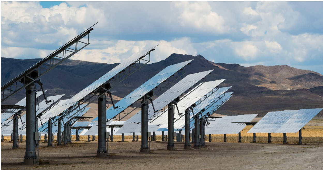
Over 10,000 tracking heliostats focus solar energy at the receiver on the 640 foot power tower at the Crescent Dunes Solar Thermal Facility, in Tonopah, NV. The facility, built with US sourced steel, glass and technology, provides more than 500,000 megawatt hours of electricity per year, available day or night through molten salt storage. Source: Dennis Schroeder / NREL
