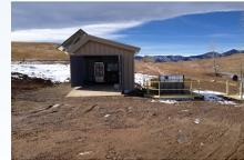
Rocky Flats Site developed a replacement for a zero-valent iron system by building a groundwater treatment component operating on solar/battery power – **saving ~3.6 MT of CO<sub>2</sub>e each year.**
