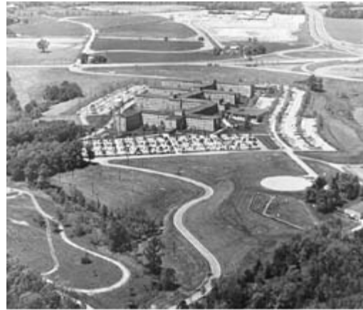
Headquarters, U.S. Atomic Energy Commission, Germantown, Maryland. A new headquarters building for the AEC was dedicated on November 8, 1957. It was determined the Germantown location (23 miles from Washington) would afford reasonable protection against blast effects of a thermonuclear weapon in the event of an attack on the Nation's capital.
