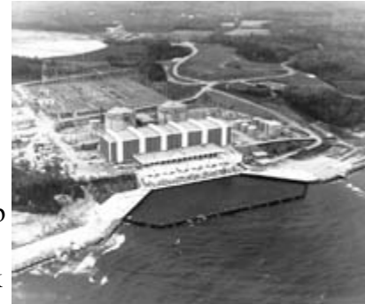
Aerial view of Baltimore Gas and Electric Company's Calvert Cliffs Nuclear Power Plant on the Chesapeake Bay near Lusby, Maryland.
