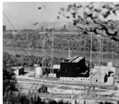
Shippingport Atomic Power Station, the Nation's first full-scale nuclear generating station.
