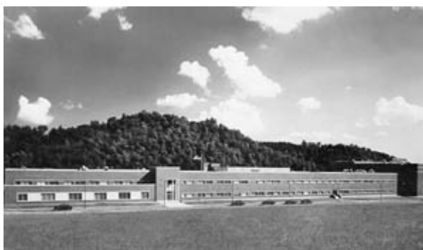
Main Research Building, Oak Ridge National Laboratory.
