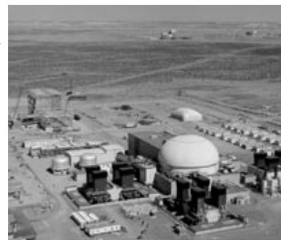
Aerial view of the Fast Flux Test Facility, Richland, Washington. The FFTF, a 400 megawatt (thermal) sodium cooled fast flux reactor, achieved full power on December 21, 1980.
