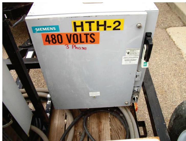
Figure 4. Typical Disconnect Switch
