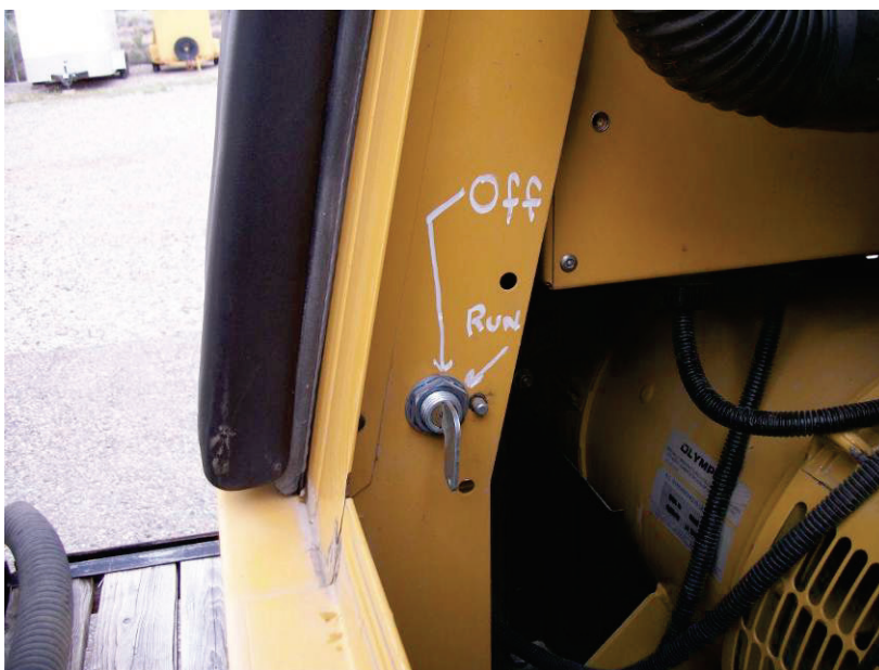
Figure 2. Battery Isolation Switch
