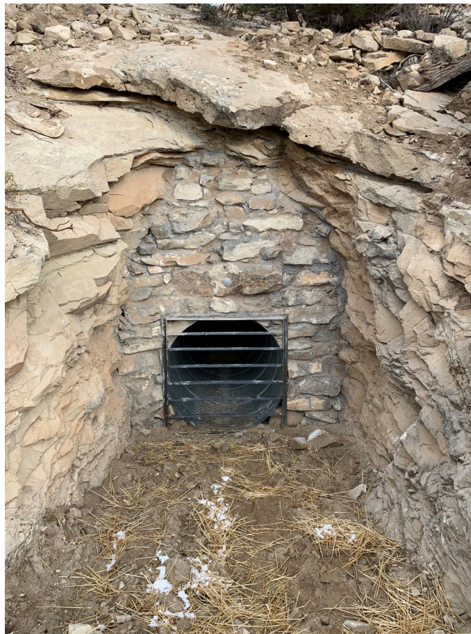
Figure 10. Adit safeguarded with bulkhead and bat-accessible grate (Klondike Basin Safeguarding Project, Photo Courtesy of DRMS)
