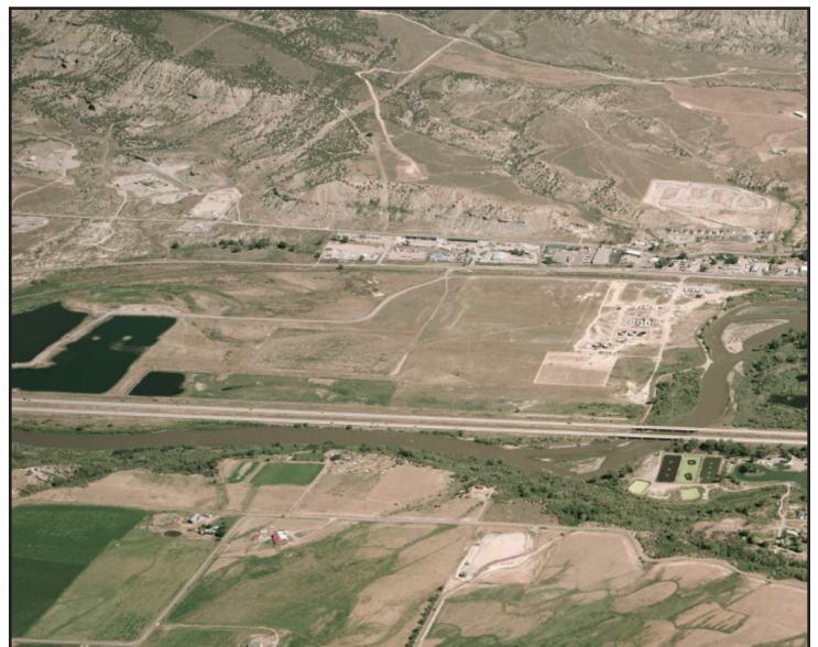
New Rifle Processing Site in 1974 (above) and 2008 (below).
