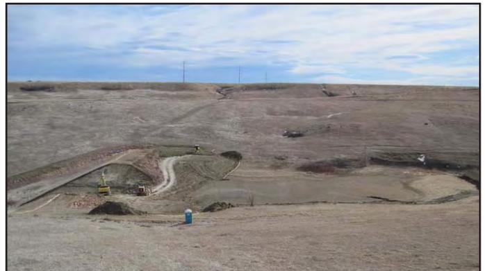
*Heavy equipment is used to excavate a notch in the dam to create a channel for surface water flow.*
