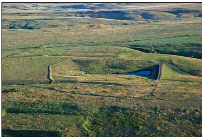
The Present Landfill Pond dam is scheduled to be breached in the fall of 2011. The dam has been operated in flow-through condition for the past several years.
