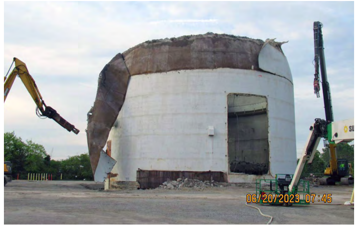
Phase 4 required elevated torch cutting the dome's steel skin, then "peeling" it away before demolishing the concrete reactor building from the top down.
