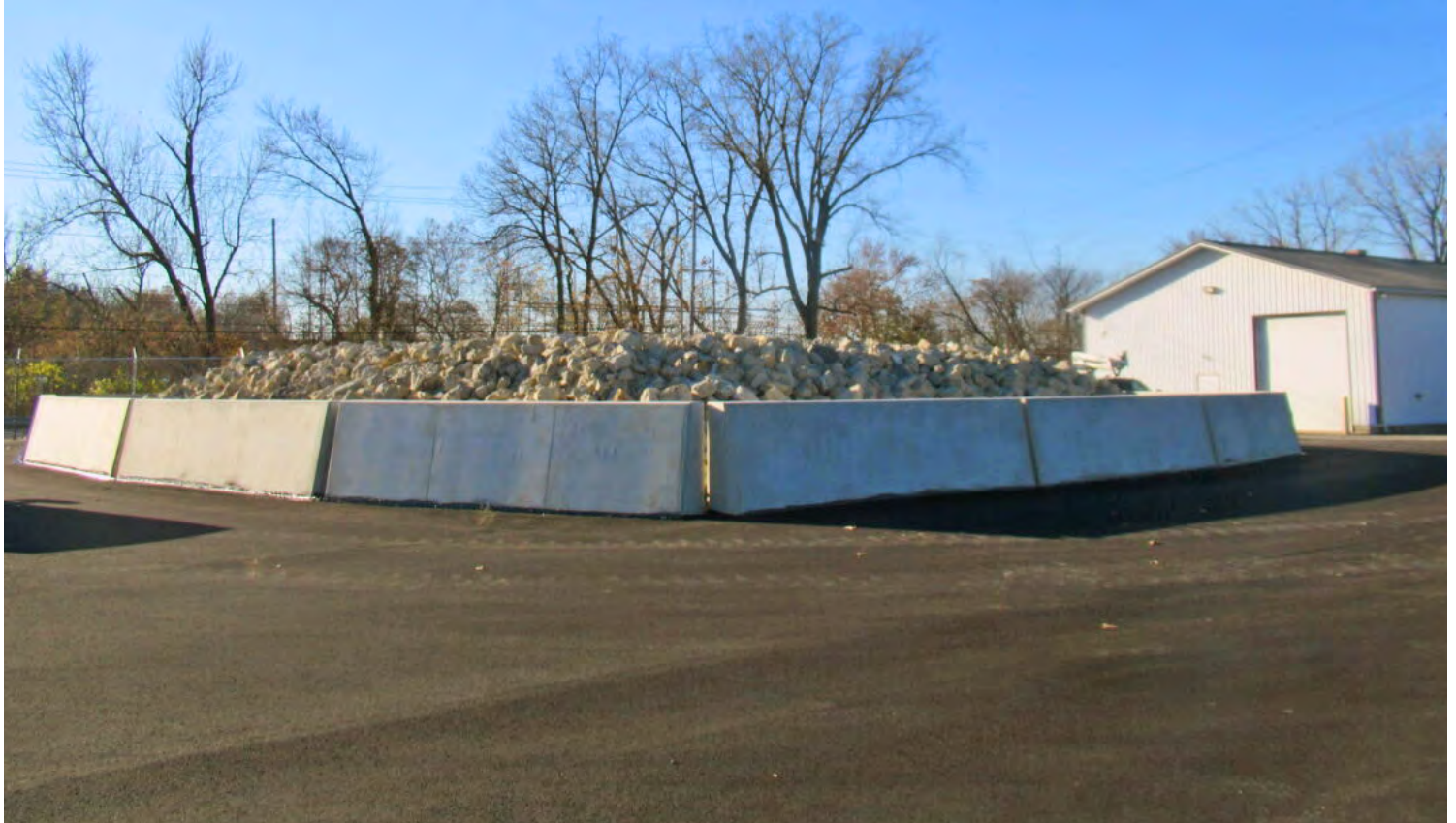
The entombment sits below grade, fully enclosed in a 10-foot-thick concrete barrier. The surface includes a vegetation barrier and loose stone cover, known as riprap, secured by heavy-duty jersey barriers. The city can use the surrounding parking lot as a laydown area.
