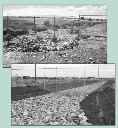
Storm damage to an outflow channel at the Shiprock, New Mexico, Disposal Site (top photograph) resulted in redesigning and repositioning the channel (bottom photograph).
