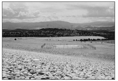
Transient drainage water is pumped from the Rifle, Colorado, Disposal Cell to an evaporation pond.
