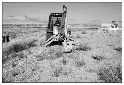
Erosion repair was necessary to protect a perimeter sign at the Green River, Utah, Disposal Site.
