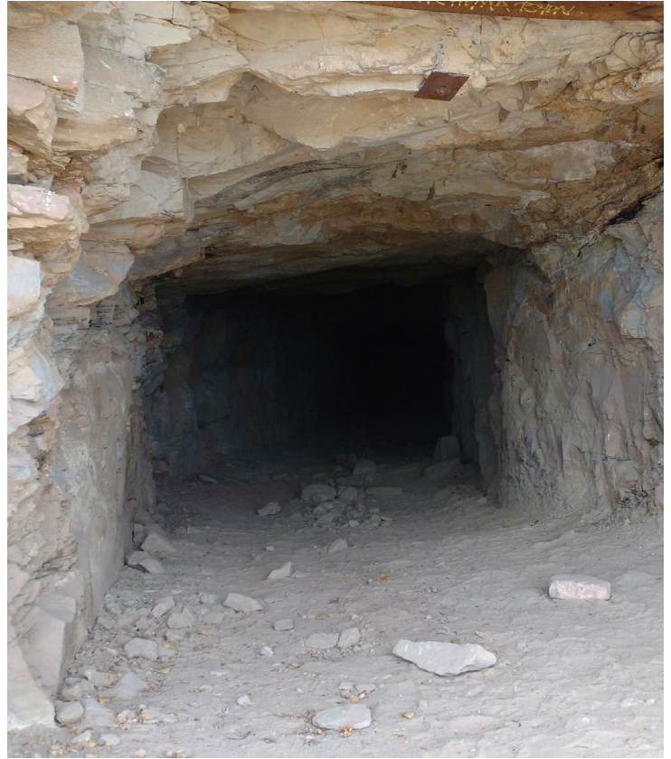
Adit at the Cedar Mine, a Small Mine Located Southeast of Moab, Utah (BLM-administered land).
