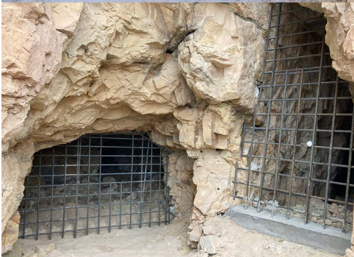
Adits at the Mucho Claims Mine, located southwest of Green River, Utah, before and after safeguarding (BLM-administered land).
