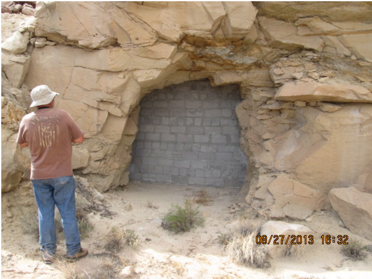
Figure 21. Mine Portal Closure by Concrete Blocks, Yellow Cat District, Utah
