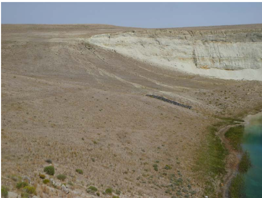
Photo 3. Recontoured and reclaimed area with channel stabilization on the north side of the Mars Group pit.
