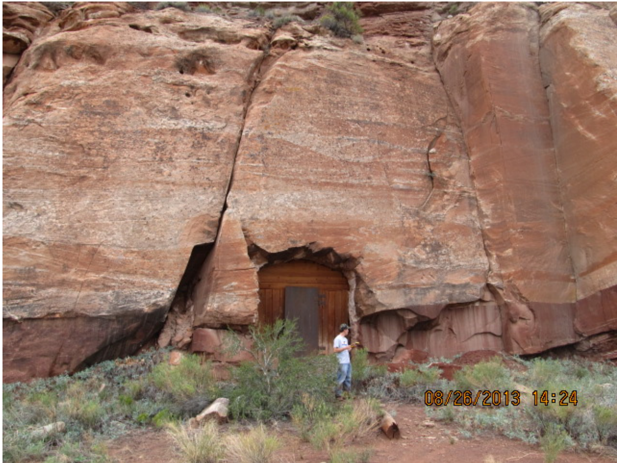
Figure 20. Mine Closure by Metal Door and Timbers. Lisbon Valley–Big Indian District, Utah
