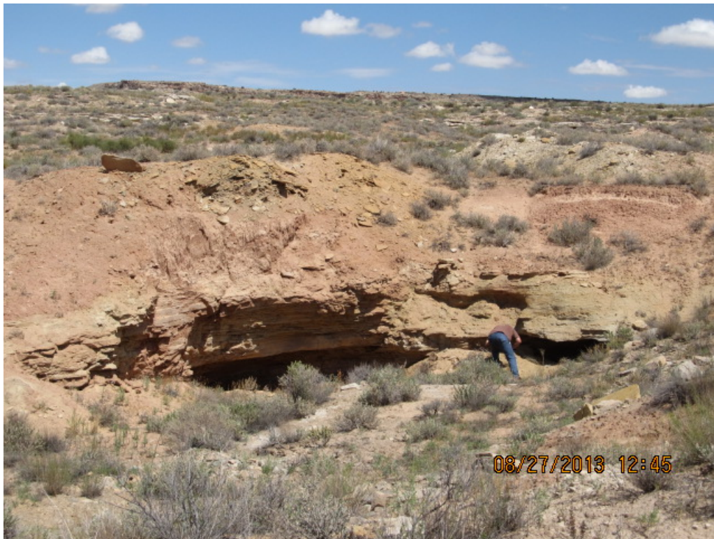
Photo 3. Paris 25 mine area alcove-type portal, looking north.
