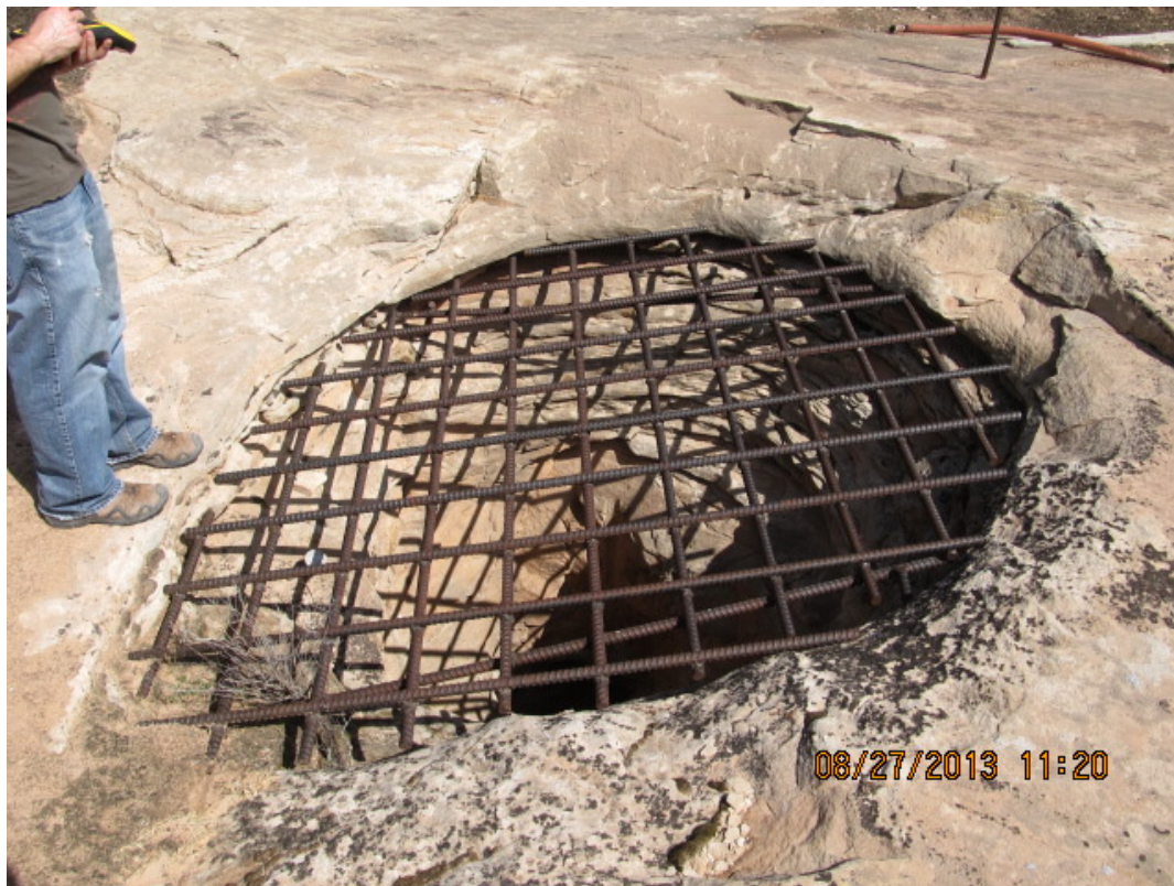
Figure 22. Top: Mine Portal Closure by Metal Gates Bottom: Mine Vent Shaft Closure with a Large Grid Rebar Typical of "Bat Gates"
