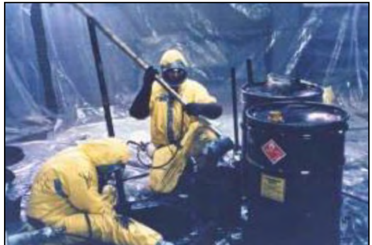
Removing sludge and placing it in drums at the Chicago North site (1987).
