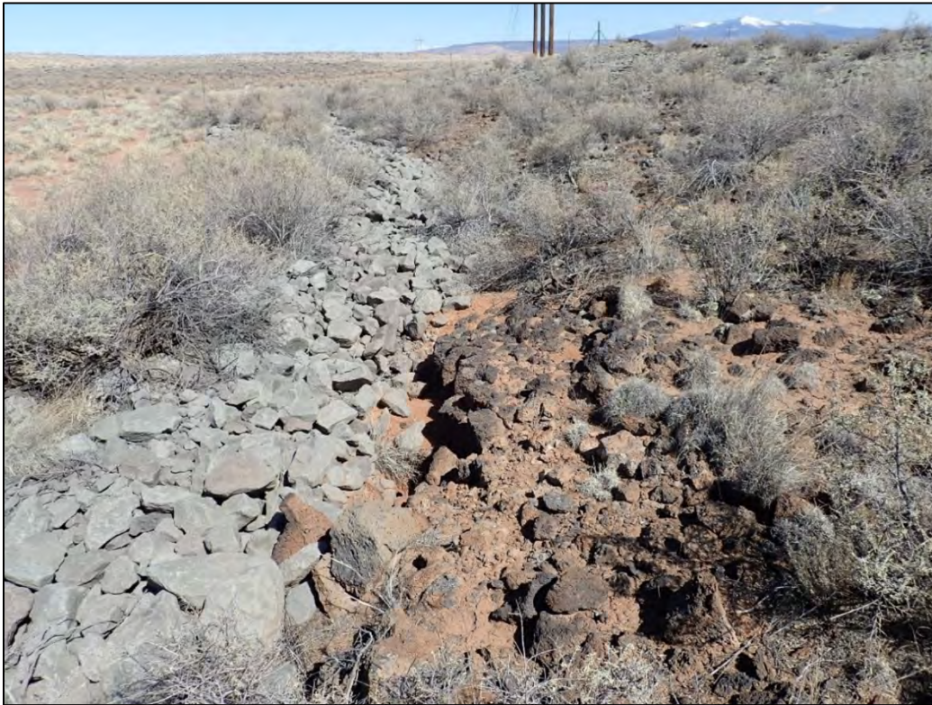
PL-23. Settlement Along Natural Basalt and Limestone Riprap Interface at East Dump
