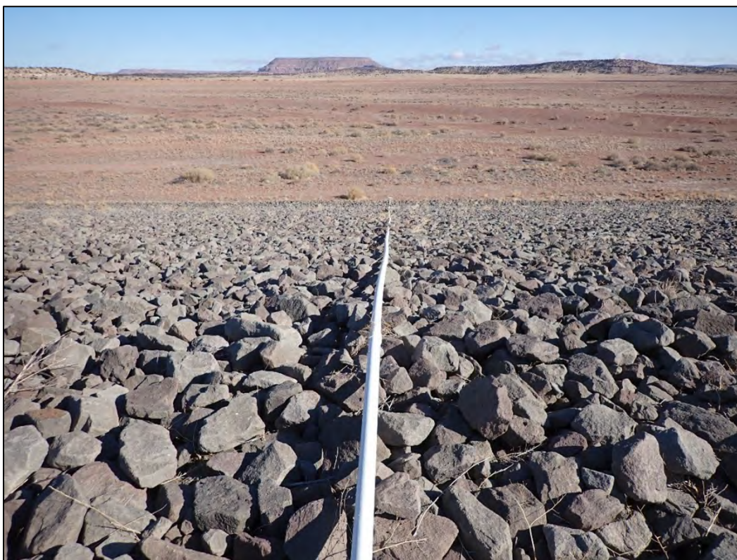
PL-16. Siphon on North Side Slope of Main Tailings Disposal Cell
