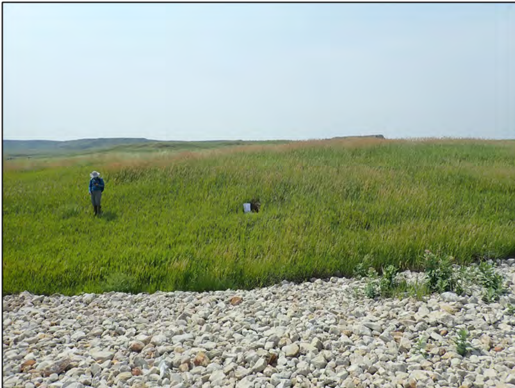
PL-8. Animal Burrow Adjacent to Toe of Armored Disposal Cell Side Slope
