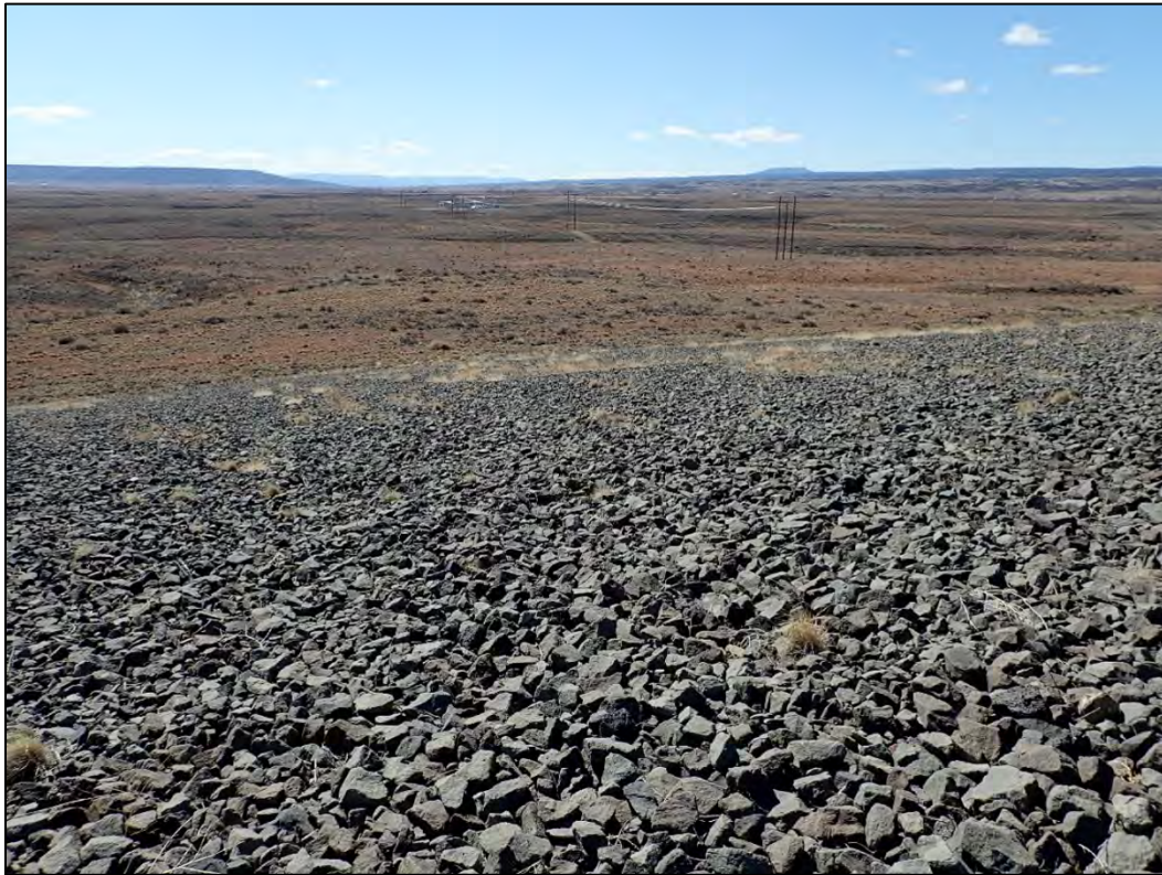
PL-17. Area of Possible Depression on Main Tailings Disposal Cell South Side Slope
