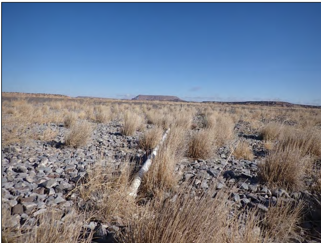
PL-15. Siphon on Top Slope of Main Tailings Disposal Cell
