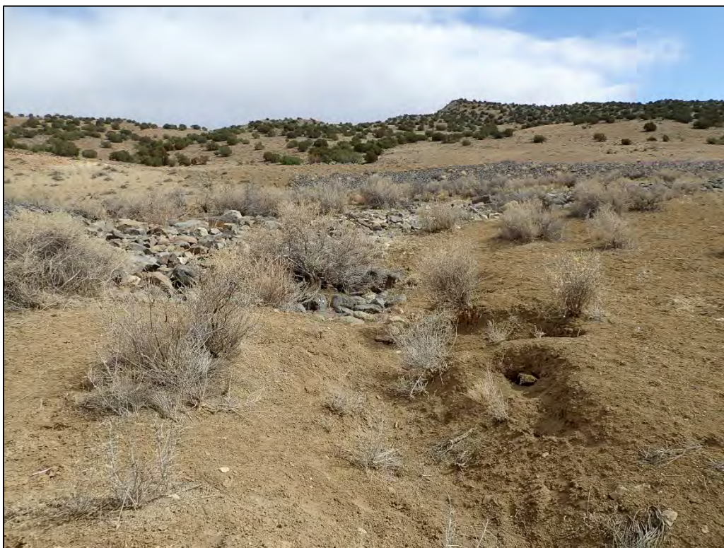
PL-18. Minor Rilling Downgradient of South Diversion Channel Cutoff Wall
