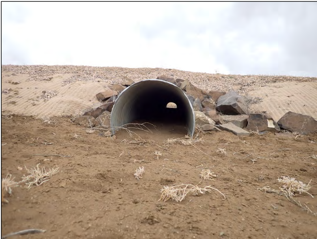
PL-2. Sedimentation in Eastern-most Culvert (Installed in 2016)
