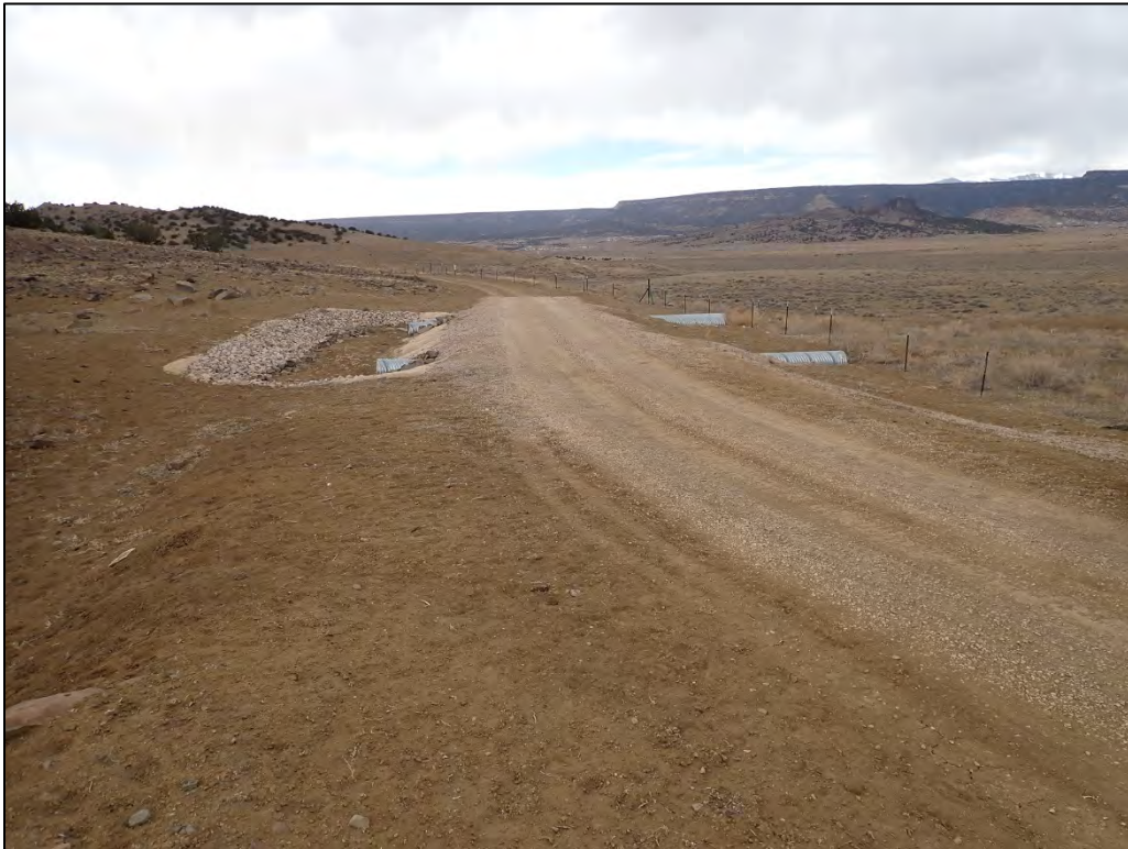
PL-1. Culverts Installed in 2016
