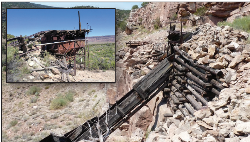
Cribbing and ore chute at the Merry Widow Mine in Colorado (main photo) and Ore Bin 4 at the Paradox 4 Mine in Colorado (inset photo).
