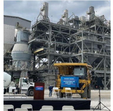
Heidelberg Cement Plant in Mitchell, Indiana
