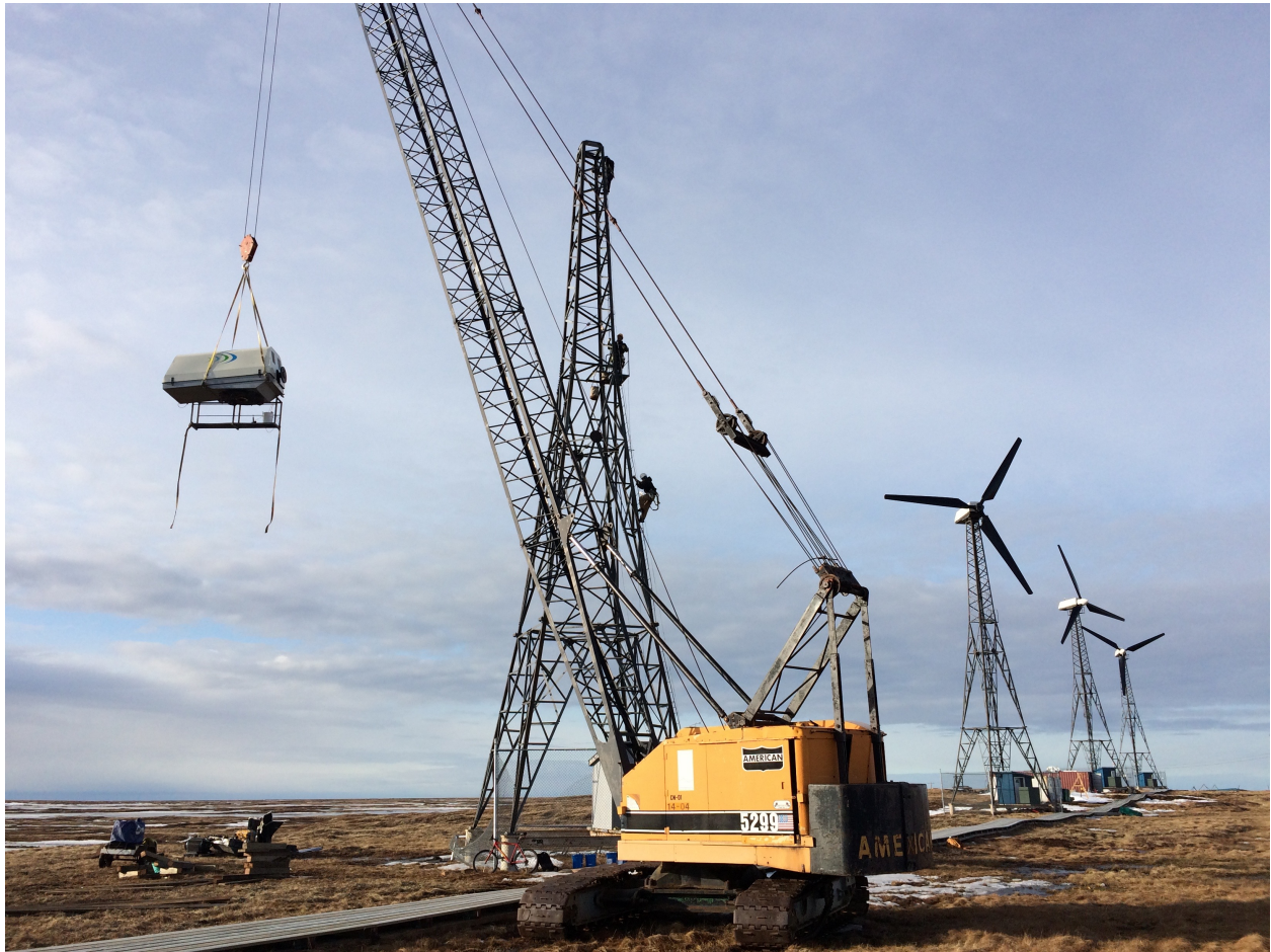
Nacelle being lifted into position
