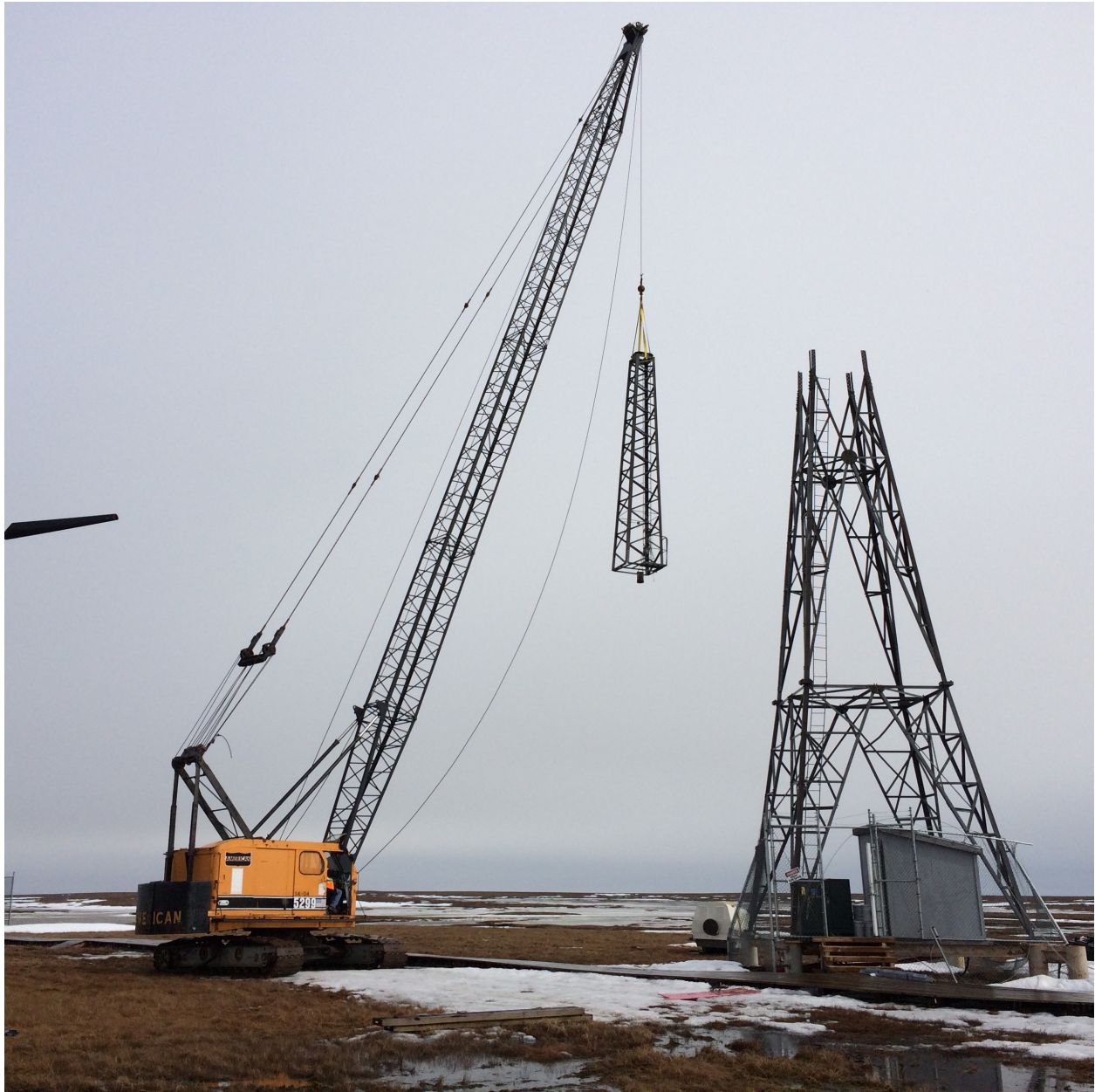
Tower repaired and being lifted into position
