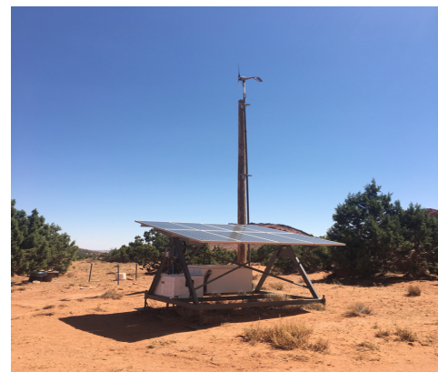
Figure 12: Navajo Tribal Utility Authority unit, 8 Module Hybrid Wind Turbine that produces 2 KWH/day (Photo Credit: Christian Gould)
