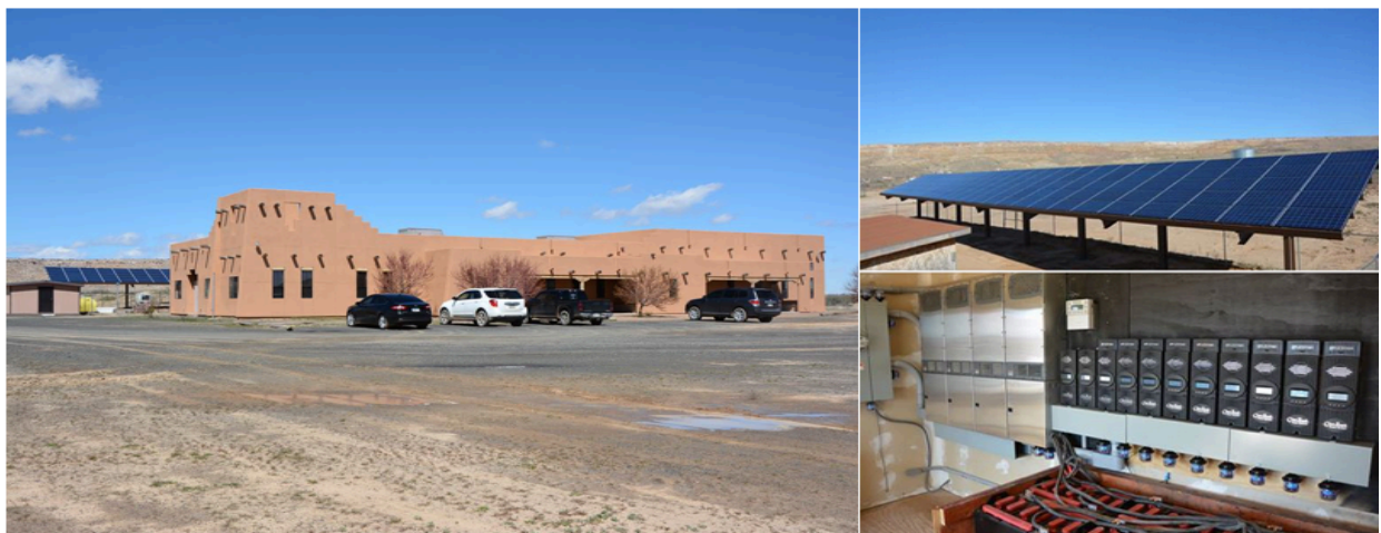
Figure 7: Hopi Tewa Community Center (Photo Credit: The Solar Exchange Arizona)
