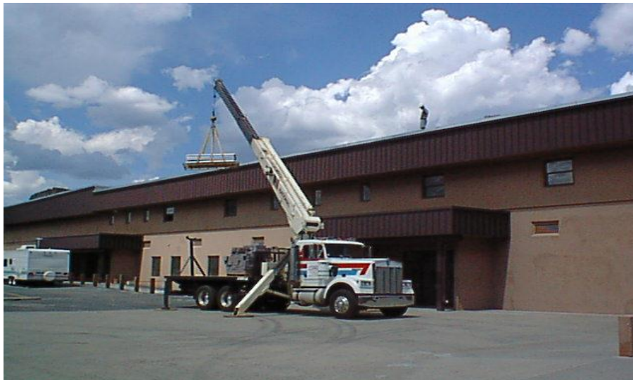
Figure – 6 Hoisting PV System material atop the Dulce High School roof.
