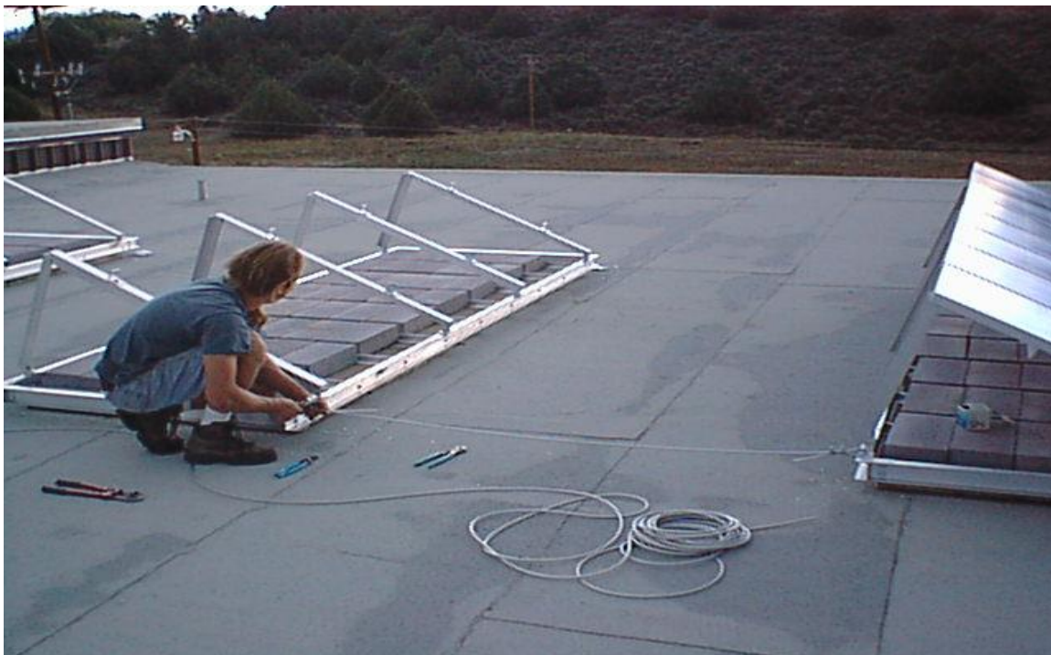
Figure – 8 Assembling racks on the Dulce High School rooftop. Concrete blocks will hold down the entire panel assembly. Four racks were assembled. The rack shown to the right is a complete assembly.
