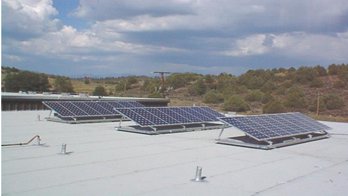
Figure – 9 Three panels of the completed PV Array are shown. The entire PV System was assembled in one day. A permit to modify the existing Dulce High Schools electrical panel was secured by Backus Electrical of Santa Fe, New Mexico.
