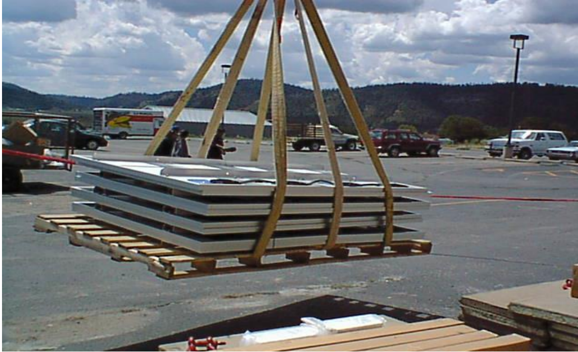
Figure – 7 PV System panels being lifted for placement onto the Dulce High School rooftop.
