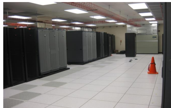
Figure 6. DC2 Lighting, and Perforated Tiles
