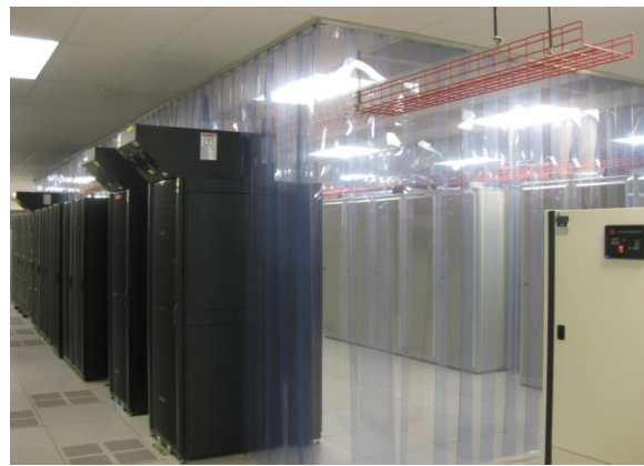
Figure 2. DC1 Hot Aisle Containment
