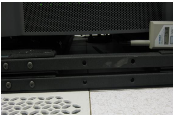
Figure 5. Air Recirculation Under the Racks
