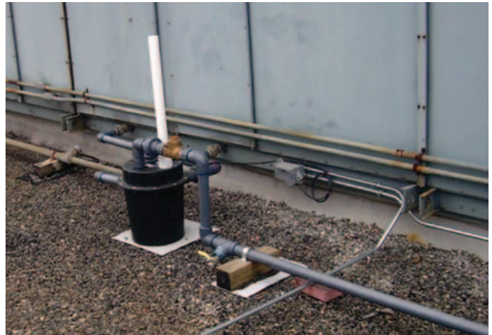
Initial piping and the condensate collector next to one air handler unit
