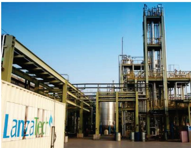
A gas fermentation facility at the Shougang Steel mill in Caofeidian, China. Commercial-scale biological gas fermentation processes are currently being deployed to convert carbon-rich gas waste streams produced through steel manufacturing into low-carbon fuels. Pioneer plants are able to produce over 45,000 tonnes of fuel per annum. | Image courtesy of LanzaTech Inc.
