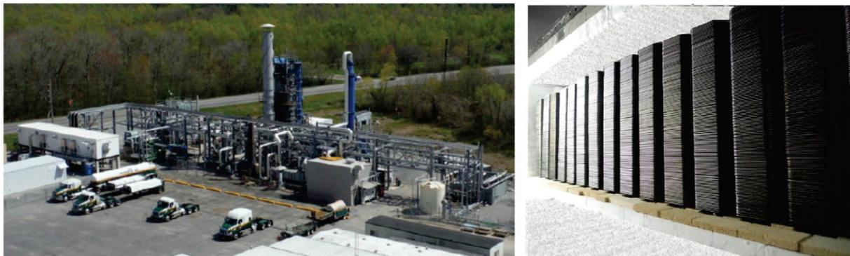
**Figure 2.11.** (a) Intermediate-scale test unit, capable of producing up to 100 ton per day of oxygen; (b) installed ion-conducting oxygen separation modules. | Reprinted from *Solid State Ion.* 288, L. L. Anderson et al., Advances in ion transport membrane technology for oxygen and syngas production, 331–337, copyright 2016, with permission from Elsevier
