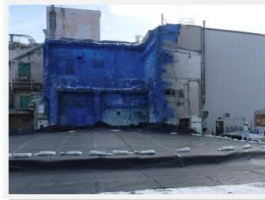
Weather protective cover installed
