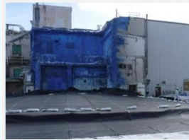
Weather protective cover installed
