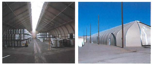
Figure 4: TRU waste storage Dome at TA-54 Area G<sup>13</sup>
