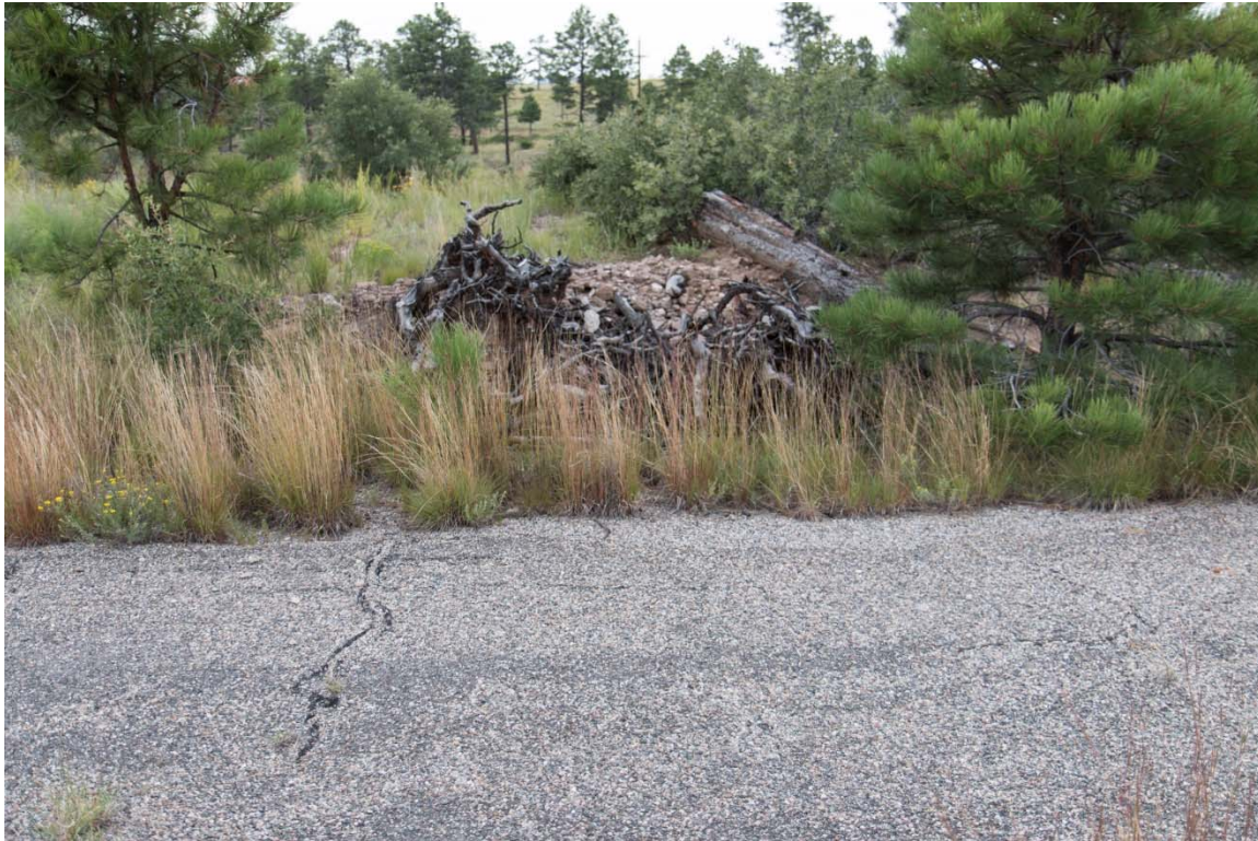
Figure I-5 Paved road north of Solid Waste Management Unit (SWMU) 15-009(b) looking southeast toward soil pile where septic tank was removed
