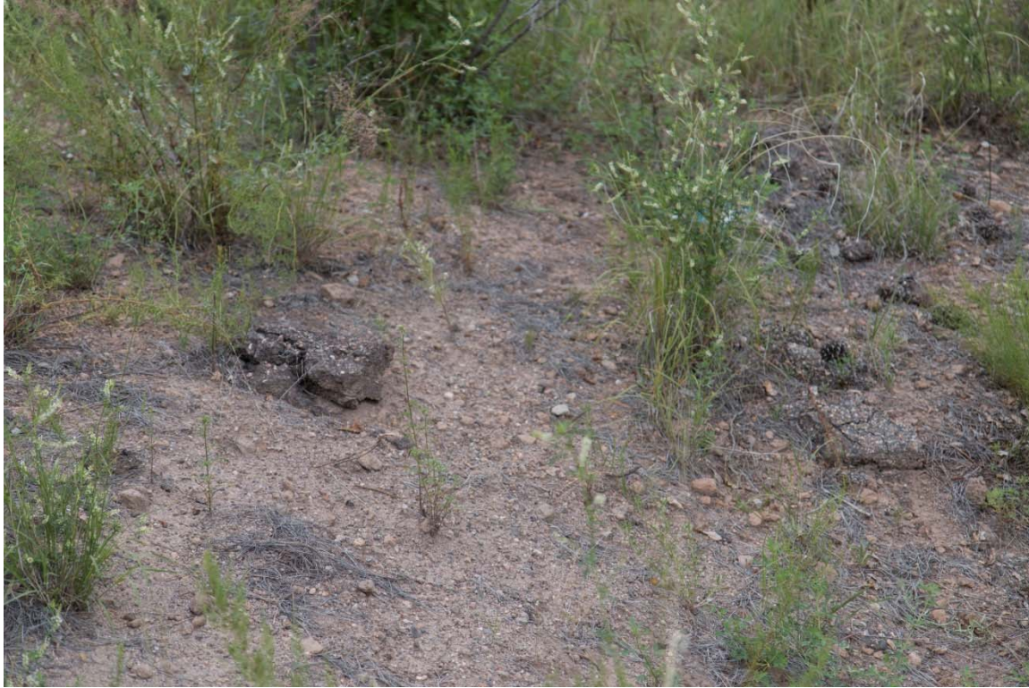
Figure I-19 Eroded asphalt debris between Potrillo Drive and SWMU 36-003(a) drain field, looking north
