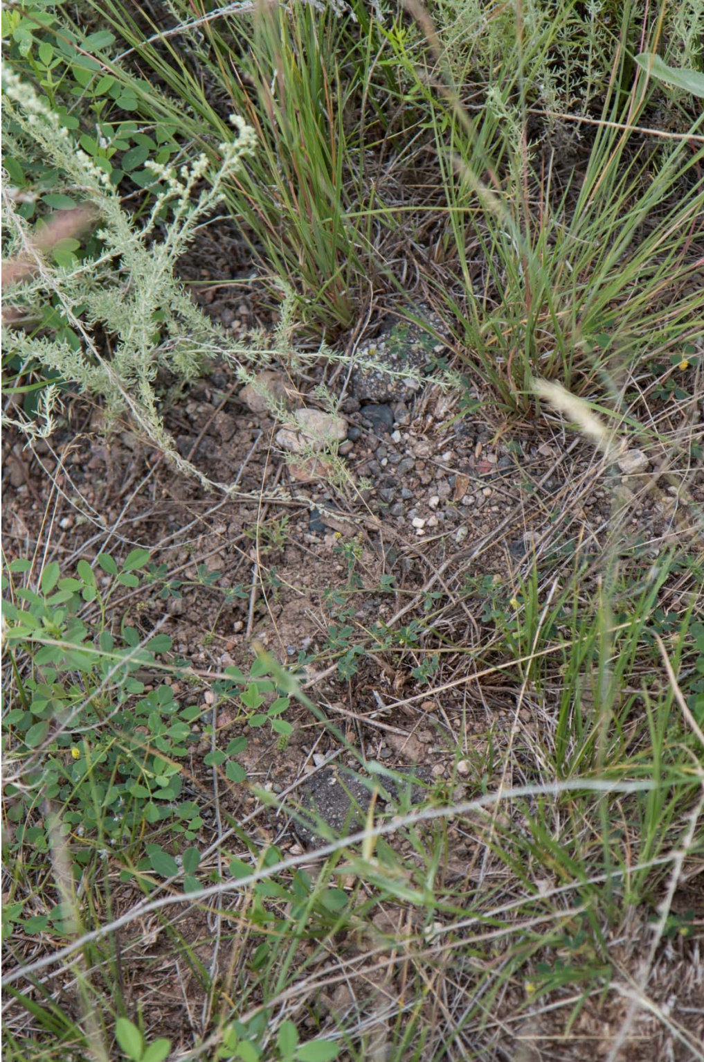
Figure I-16 Asphalt debris in drainage below AOC 15-014(h)
