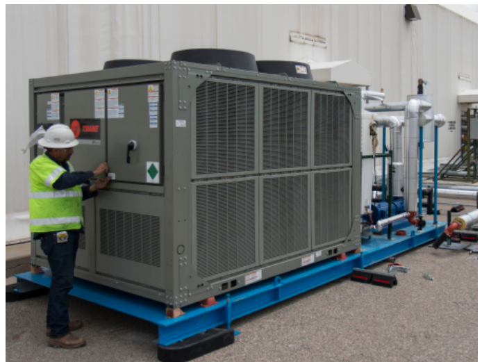
A 40-ton chiller provides supplemental cooling for the RNS drums inside the PermaCon.
