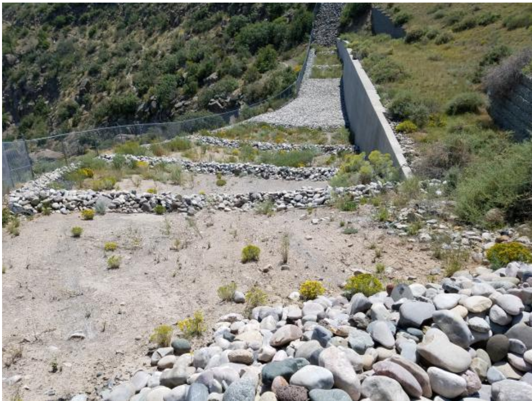
Picture 26. Rock Check Dams - Erosion Control East End of Landfill
