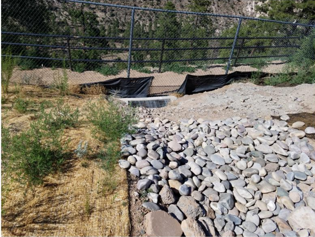
Picture 9. New Drop Inlet Structure Installed by Los Alamos County North of New Hangar Pad
