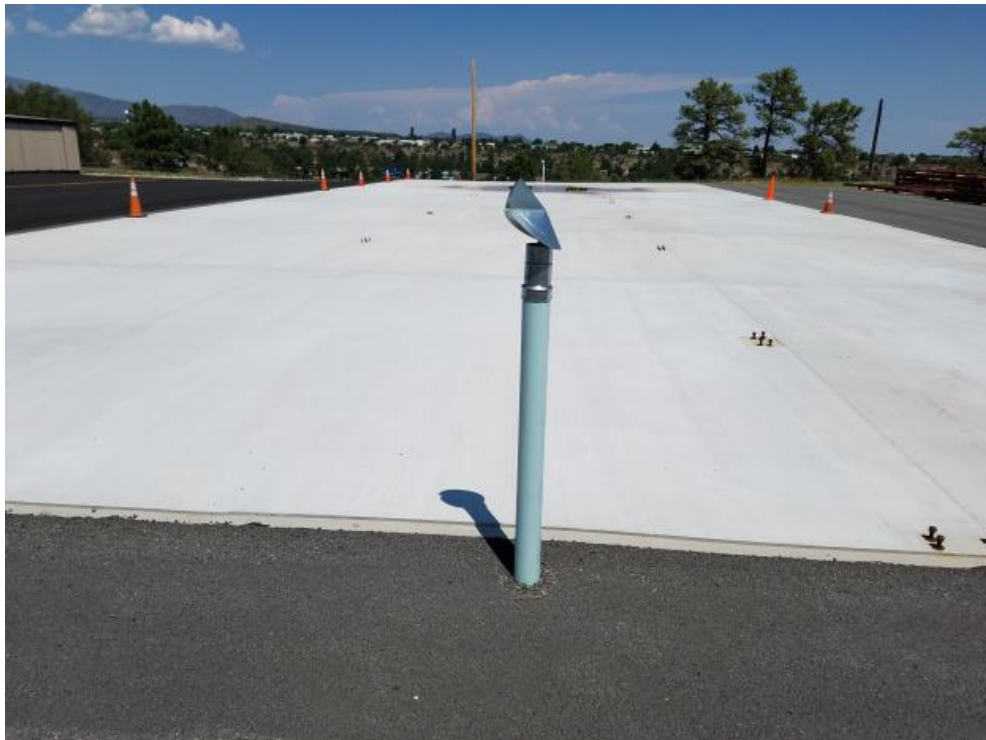
Picture 2. Methane Monitoring Port - West of Landfill
