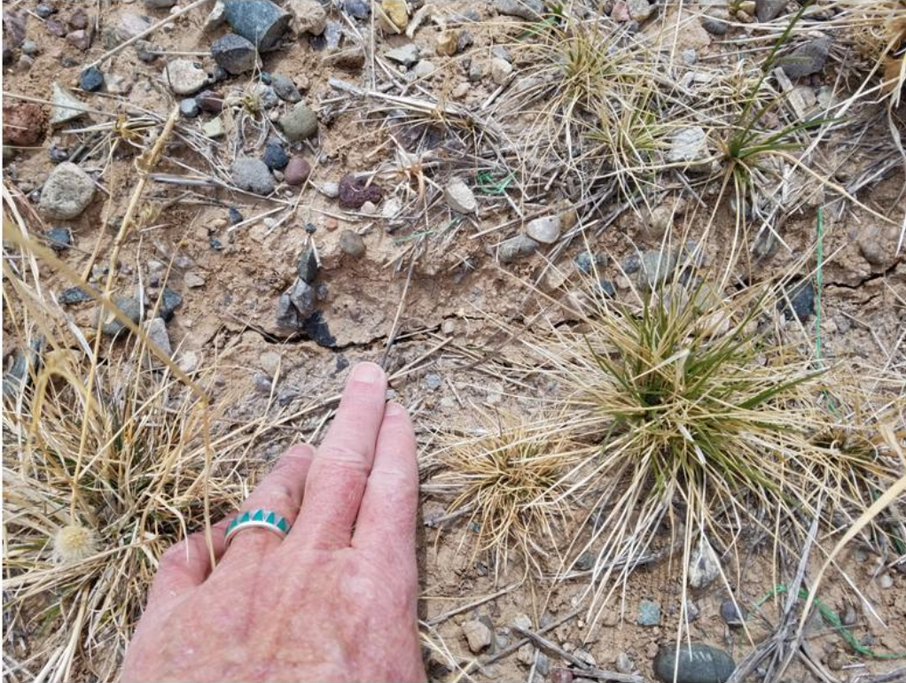
Picture 19. Surface Tension Crack – North Slope / Eastern Half of Landfill
