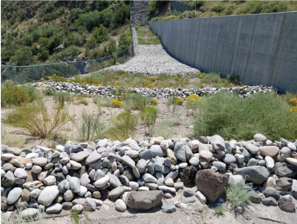
Picture 25. Concrete Retaining Wall - NE End of Landfill
