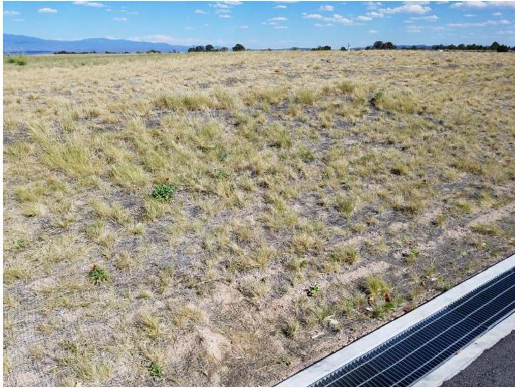
Picture 5. West Slope End of Landfill
