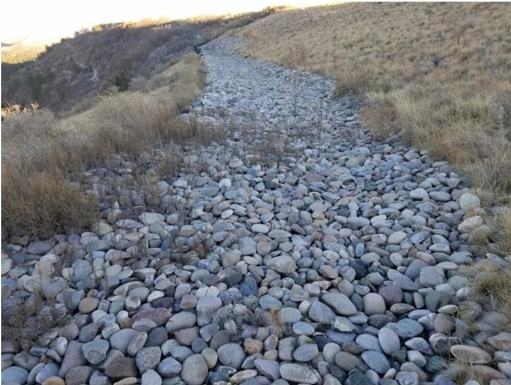
Picture 18. SE Berm - Adjacent to Airport Taxiway
