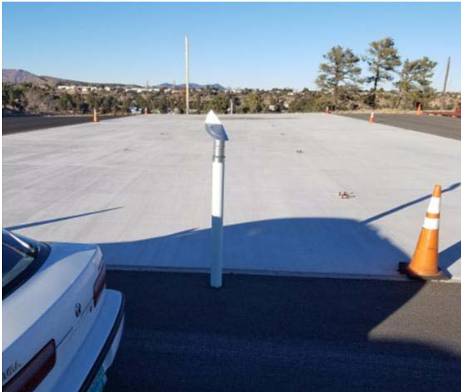
Picture 2. Methane Monitoring Port - West of Landfill
