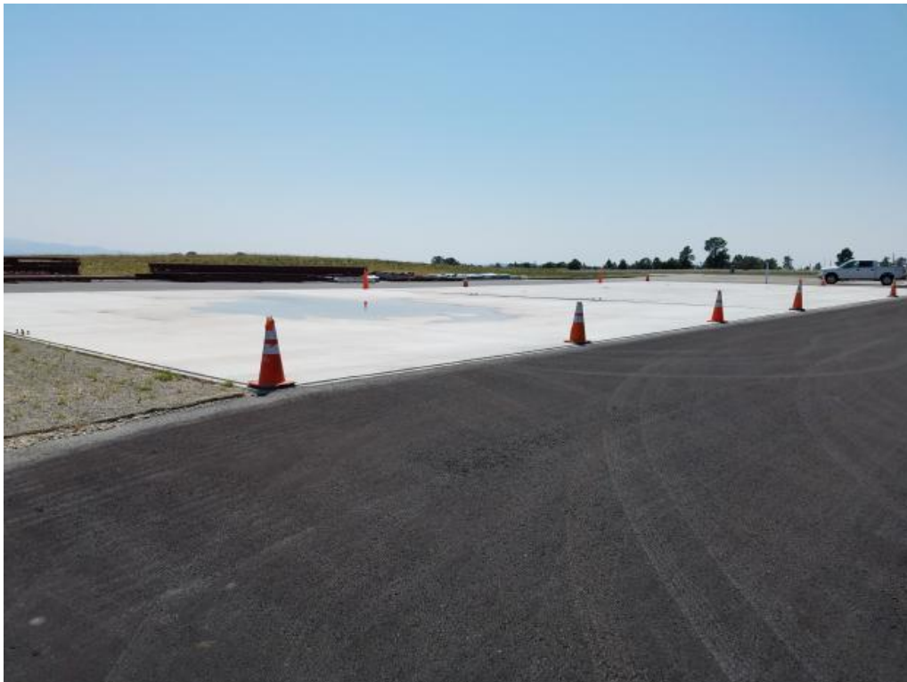
Picture 8. New Asphalt and Concrete Hangar Pad - West of Landfill
