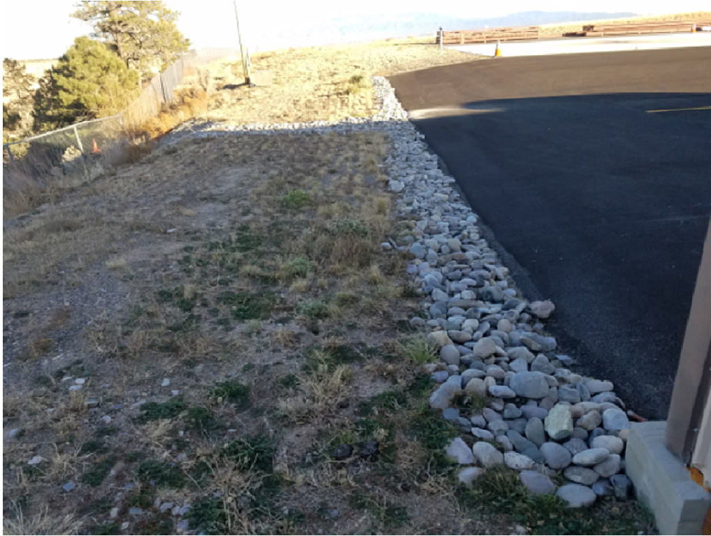
Picture 9. Reseeded Disturbed Area North of New Hangar Pad
