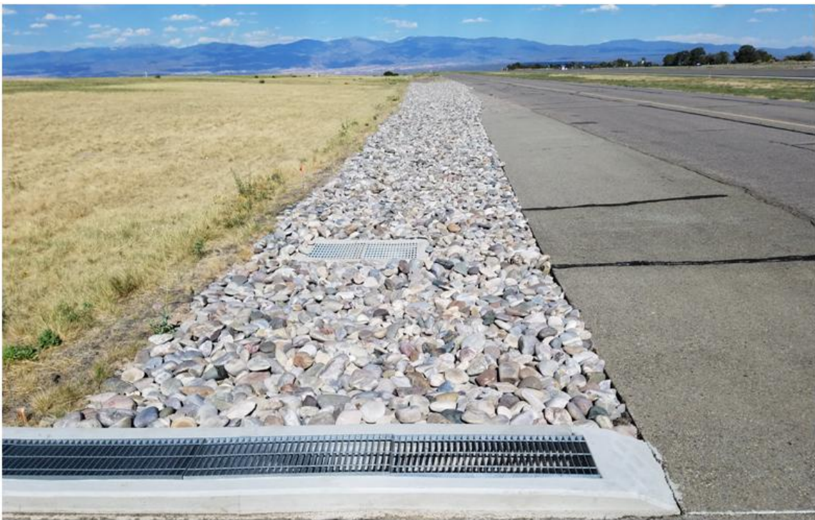
Picture 12. Drainage Channel - South Perimeter of ET Cover
