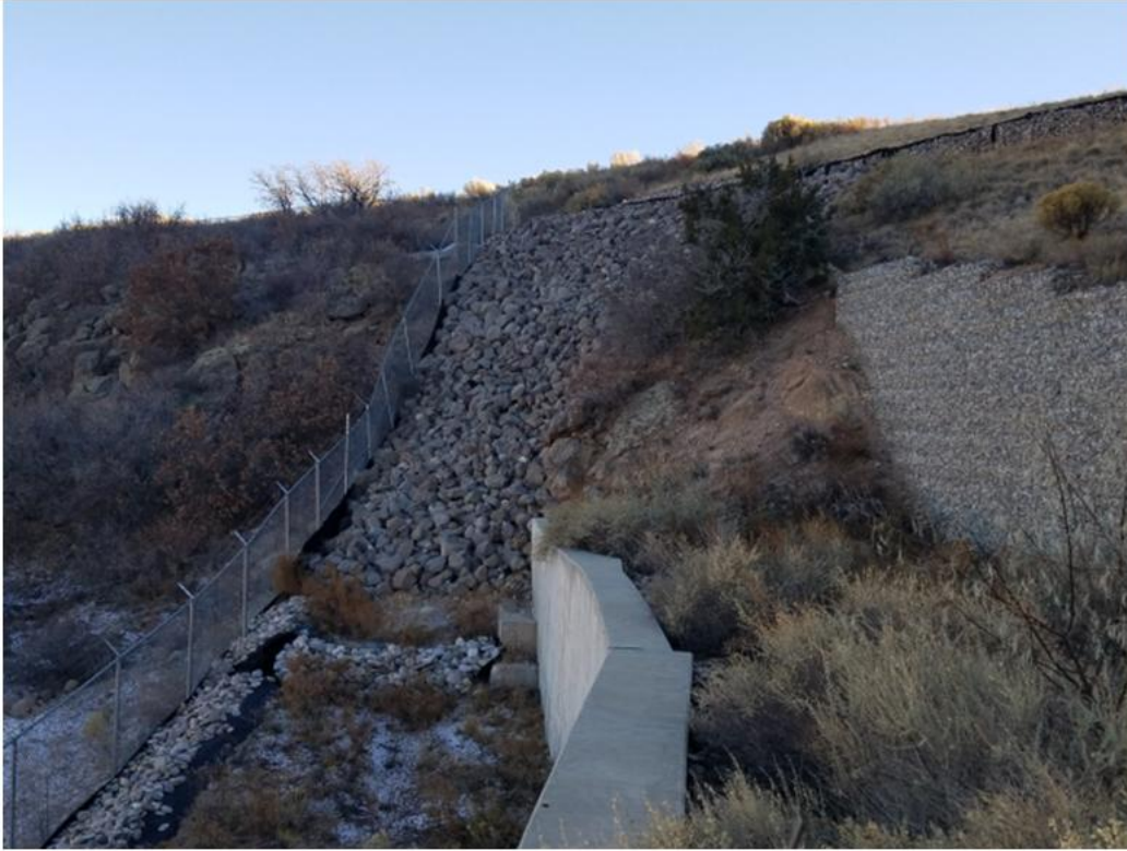
Picture 23. Large Rip Rap Slope - East End of Landfill Site
