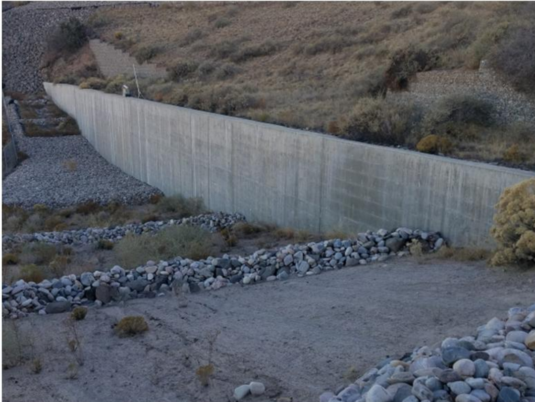
Picture 24. Concrete Retaining Wall - East End of Landfill
