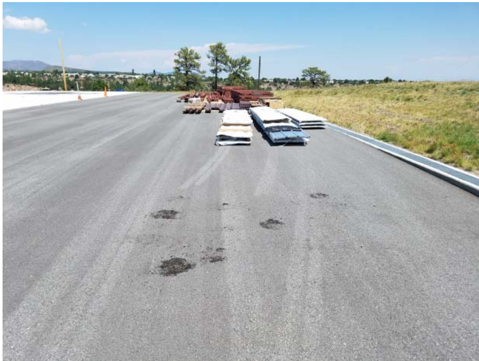
Picture 28. Materials Stockpiled for Construction of New Hangar West of Landfill
