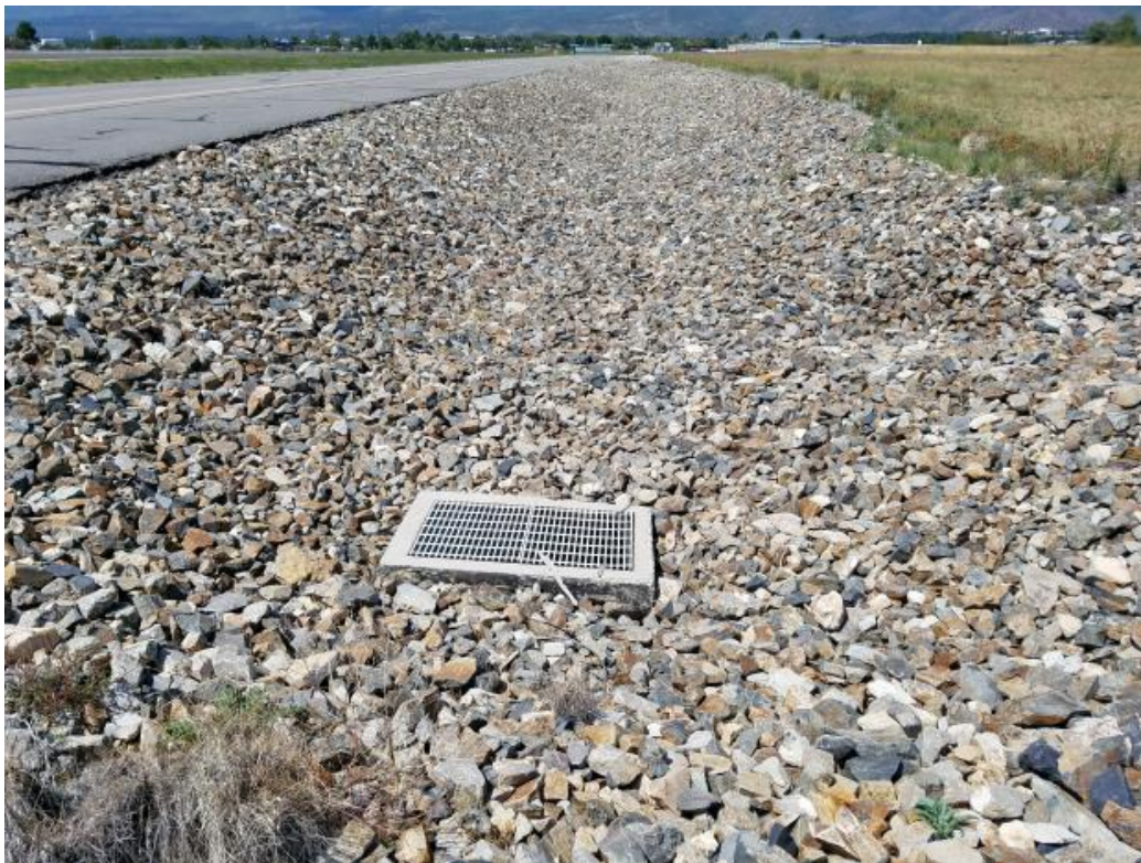
Picture 12. Drainage Channel - South Perimeter of ET Cover
