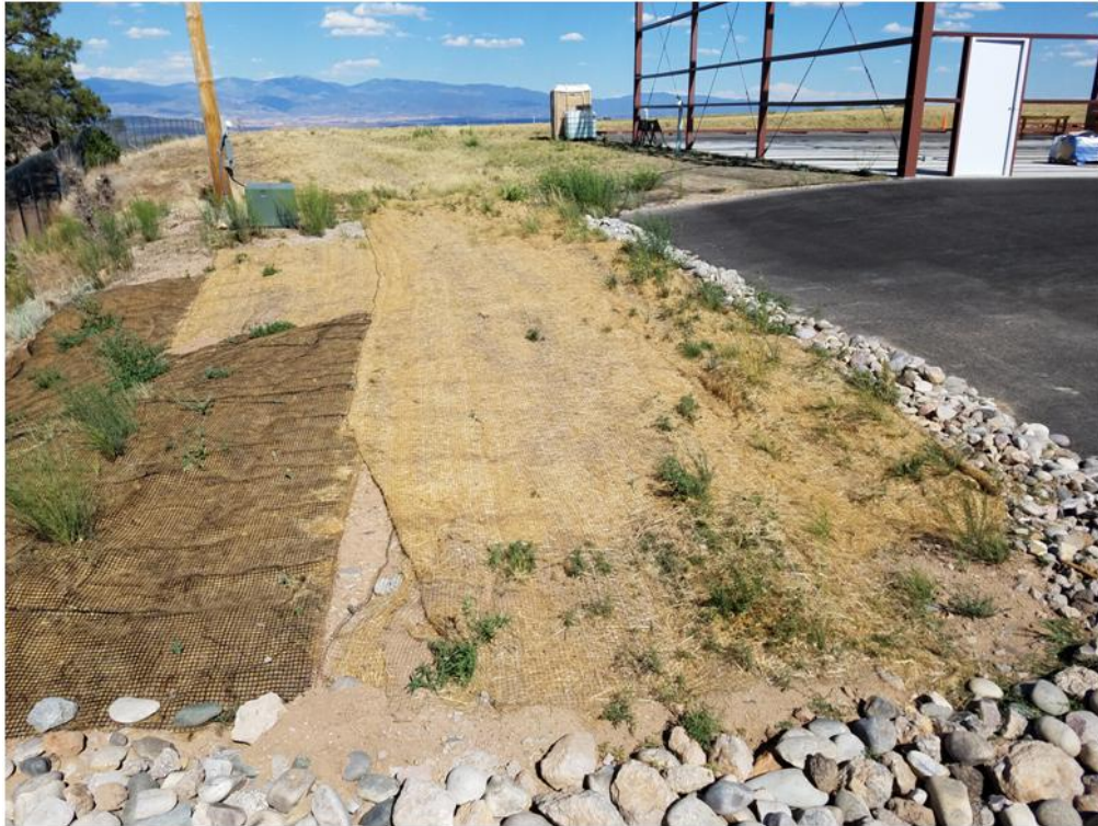
Picture 7. Recent Placement of Erosion Matting by Los Alamos County North of New Hangar Pad
