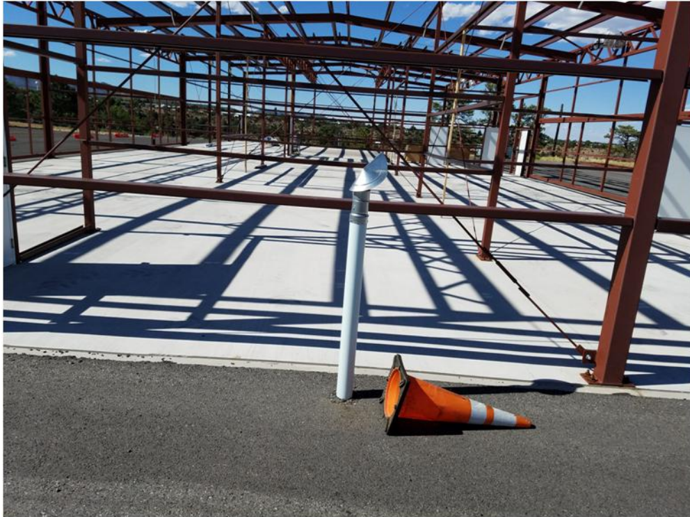
Picture 2. Methane Monitoring Port - West of Landfill
