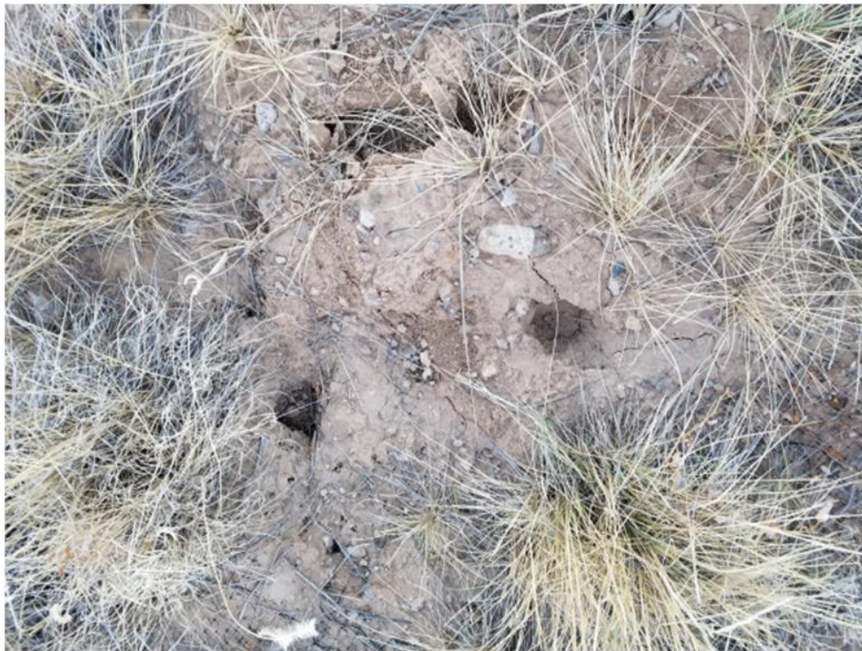
Picture 28. Burrow Holes on Side Slope of Older Landfill Cover
