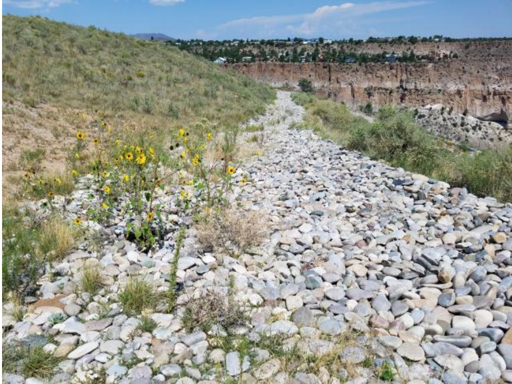
Picture 19. NE Berm - Side Slope of Landfill
