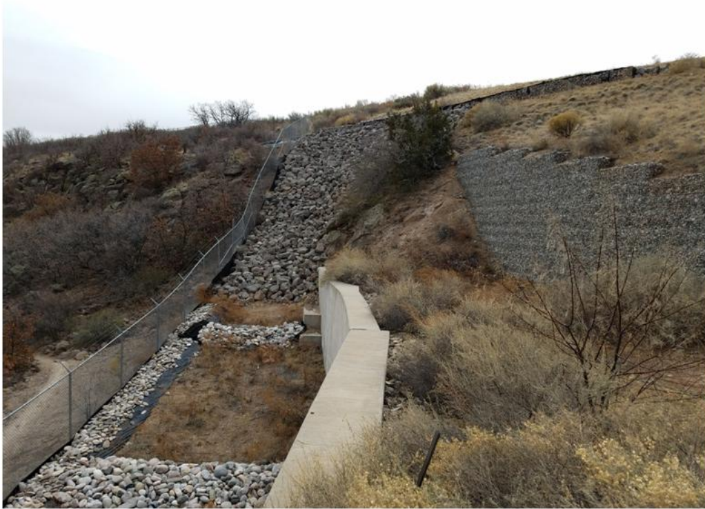
Picture 23. Large Rip Rap Slope and Gabion Retainment Wall - East End of Landfill Site
