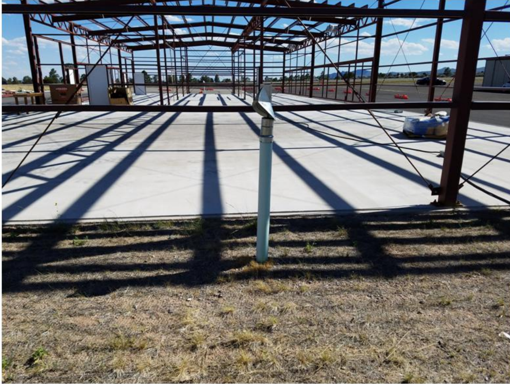
Picture 3. Methane Monitoring Port - North of New Hangar Pad
