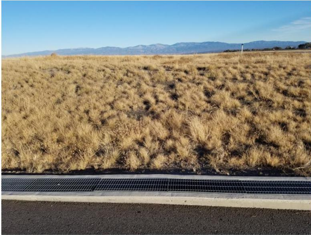
Picture 5. West Slope End of Landfill
