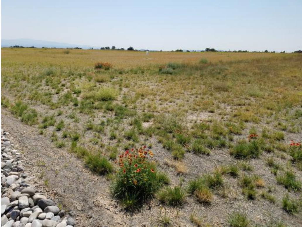
Picture 1. Cover Southeast View
