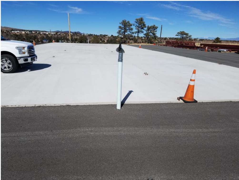
Picture 2. Methane Monitoring Port - West of Landfill
