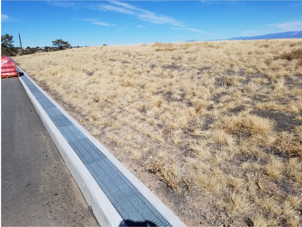
Picture 5. West Slope End of Landfill
