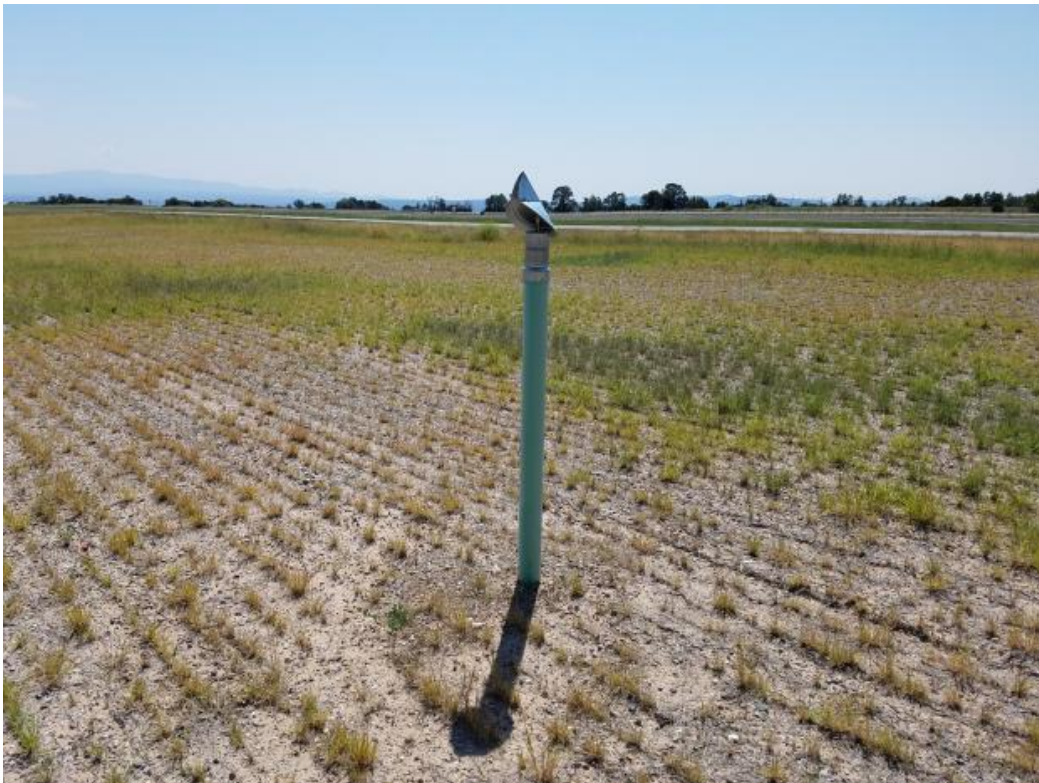
Picture 4. Methane Monitoring Port - South Slope of Landfill
