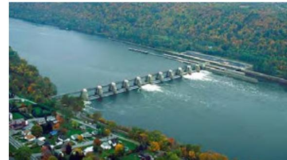
Ranking 24th in the Oak Ridge survey of potential hydropower sites is the non-powered Montgomery Locks & Dam, spanning the Ohio River near Monaca, Pennsylvania. Built in the 1930s to increase the navigational depth of a shallow part of the river, this site has the potential to generate nearly 100 MW of electricity.
