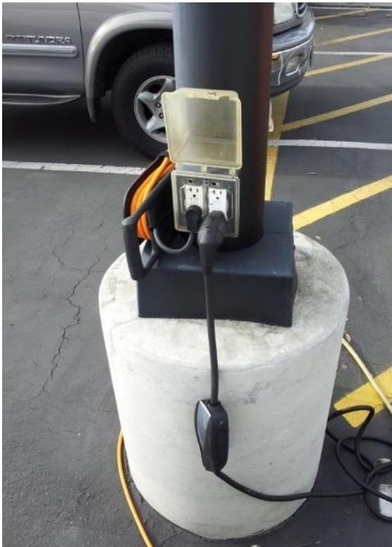
Photo 9. Level 1 charging receptacles can be installed on parking lot lamp posts. Photo from Idaho National Laboratory.
