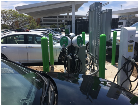
Charging Island Side View Two chargers per pedestal – 4 total for 3FCA and 1 Honda PHEV
