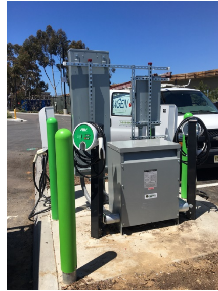
Charging Island Back Side Are two chargers located on each side of 75kVA transformer – See Side View
