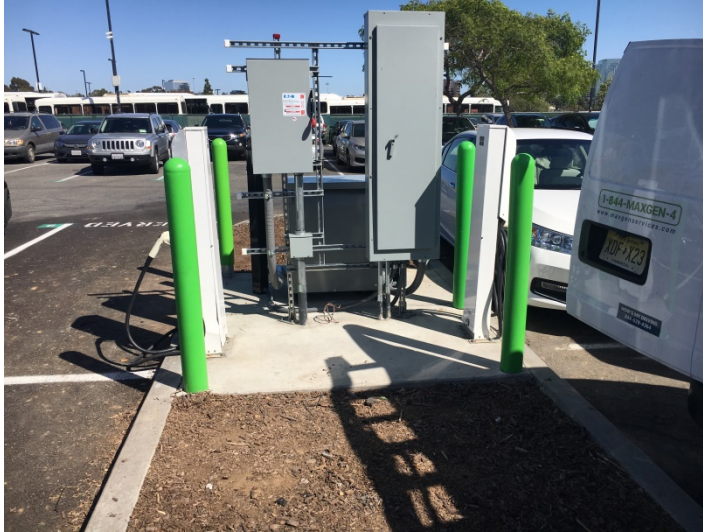
Charging Island Front Side 400A Distribution Panel and Disconnect Box
