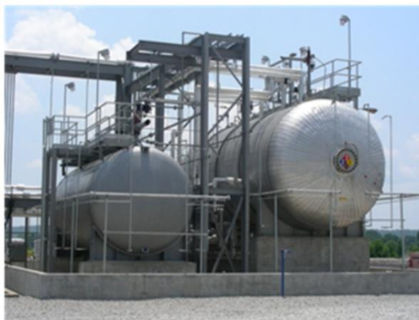
Figure II - 77: Xylene Tanks (FutureFuel Chemical Company).
