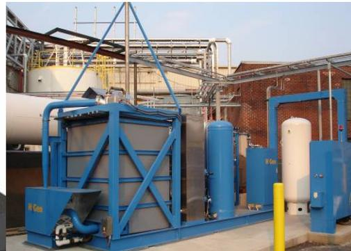
Figure 2: H2 Gen Innovations 565 kg / day steam methane reformer actual installation
