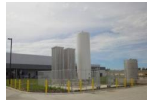
Acetone Tank and Nitrogen Tank
