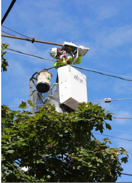
Figure 4. Installation of LED cobra head replacement luminaire in Portland, OR, July 2015
