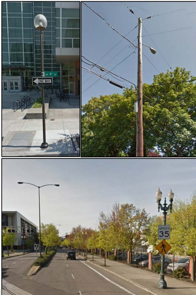
Figure 1. Sample of street/area lights and poles in Portland, OR
