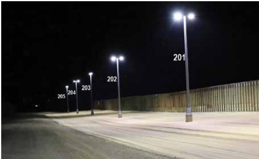
This photo was taken looking east from the area near pole 201 in September 2016. The second-generation luminaires installed in September 2016 as part of the full installation are on poles 201 and 202. The thermocoupled second-generation luminaires installed in September 2015 are on pole 204. The first-generation luminaires installed in February 2014 are on poles 203 and 205. Visible in this photo is a cooler color of sand near poles 201 and 202, and a warmer color of sand farther from the poles. This photo also shows the darkness surrounding pole 203 due to the depreciated output of its luminaires; the area around Pole 205 is relatively dark for the same reason, but also because it is the last pole in this 7.2-mile stretch of border east of the POE.
