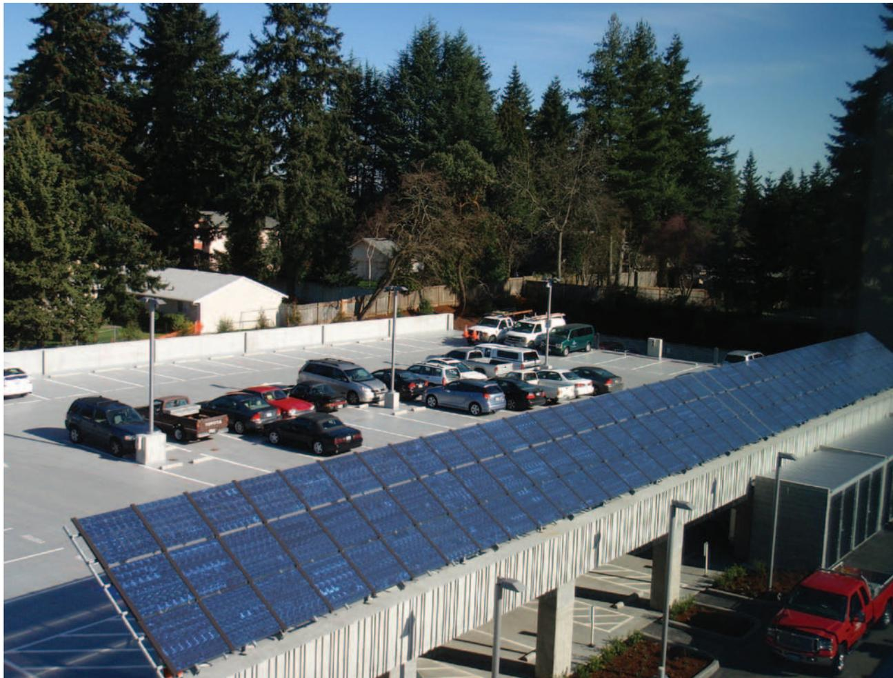
*The City of Shoreline, Washington, installed a 20.2 kW solar electric system on top of the City Hall parking garage. The system uses Washington-made solar modules from Marysville-based Silicon Energy. (City of Seattle/PIX18074)*
