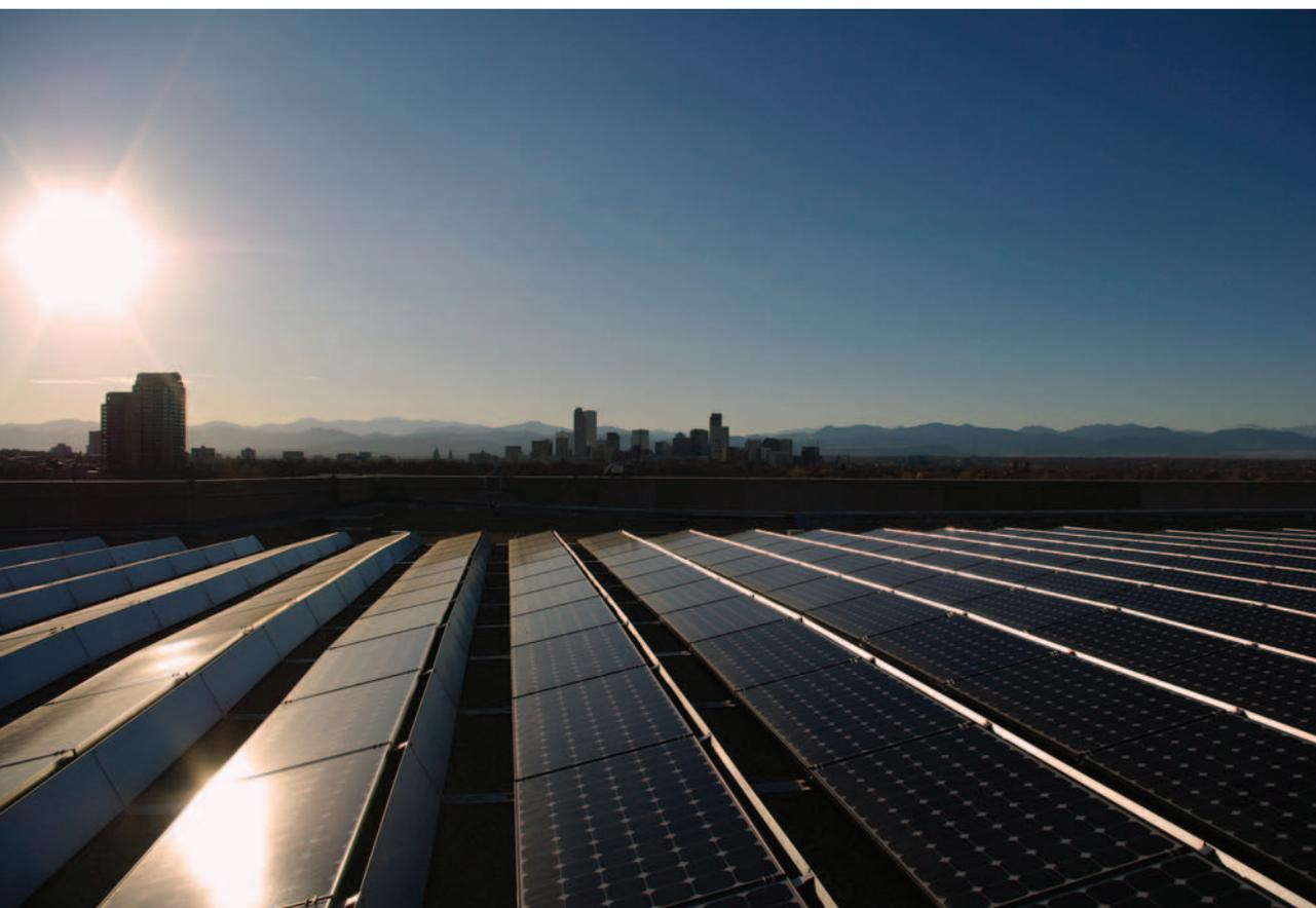
*This PV array has 465 solar panels split between roofs on the southeast and southwest wings of the Denver Museum of Nature and Science. The installation was made possible through a collaboration of Hybrid Energy Group, Partnership for Sustainability, Xcel Energy, and Namasté Solar Electric. (Denver Museum of Nature and Science / PIX18045)*
