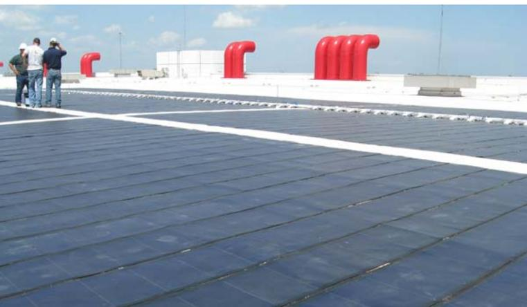
This thin film PV array is mounted on the roof of Houston's George R. Brown Convention Center. *Photo from City of Houston, NREL/PIX 19379*
