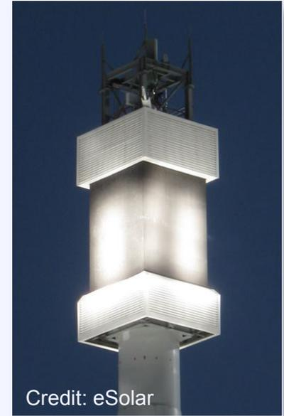
*Improved selective absorber coatings for receivers must maintain high absorptance in the solar spectrum but lower emittance in the infrared spectrum. It must also be stable in air, easily applied at large scales, cost effective, and survive thousands of heating and cooling cycles*
