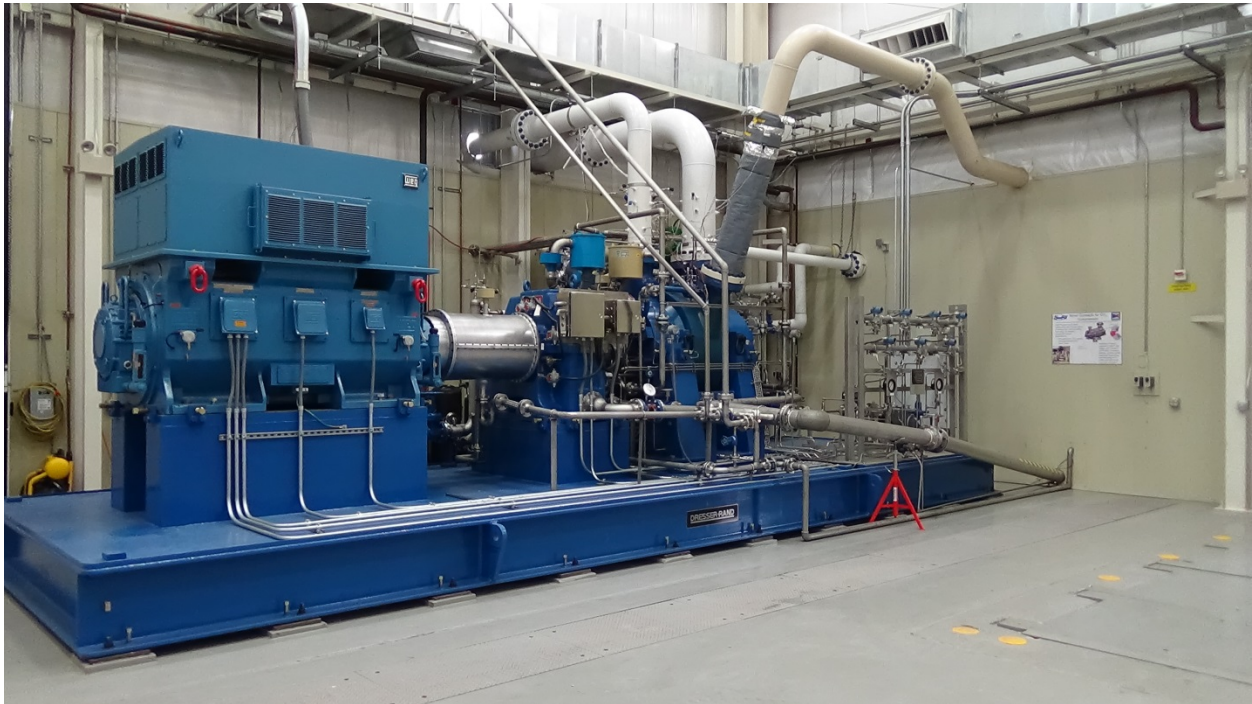
Figure 3-12. Dresser Rand Research Compressor
