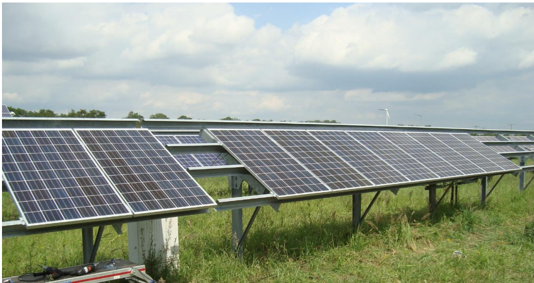
Figure 19: Installation of Direct Wafer Modules for Field Monitoring in Germany
