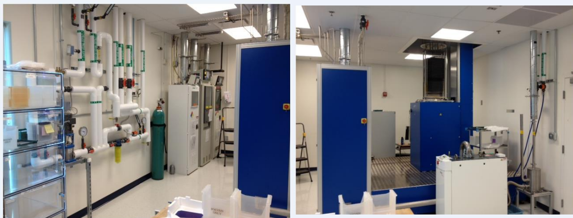
Figure 8: PECVD SiN x system (right) and gas cabinets and cooling water system (left).
