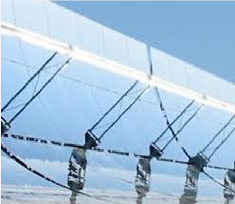
RioGlass in Surprise, Az makes the trough reflectors for Solana 300 MW CSP – one every 20s, 24/7
