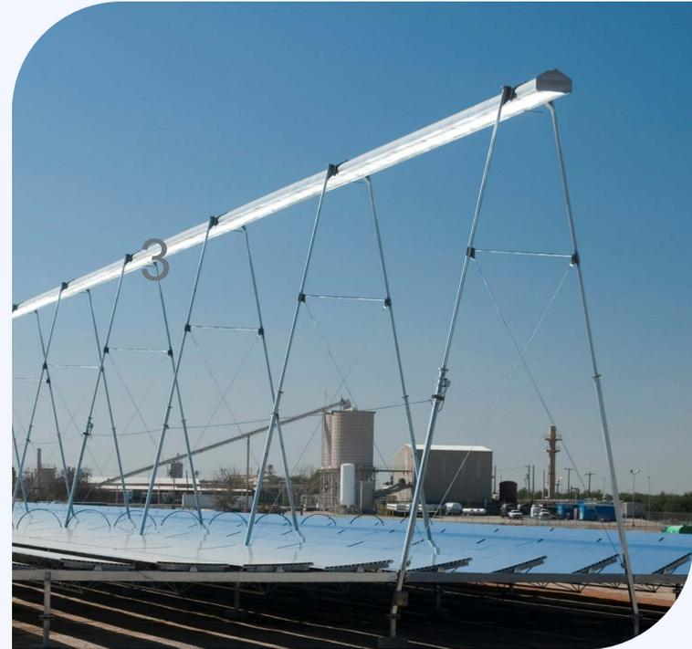
Tucson Electric Power is installing linear Fresnel glass reflectors for Ariva CSP steam boost plant
