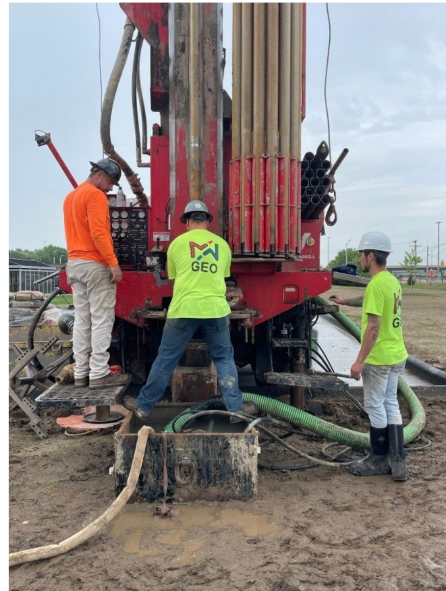
Drilling a test borehole at Detroit Arsenal SOURCE: U.S. Army. Photo courtesy Shannon Bergt.
