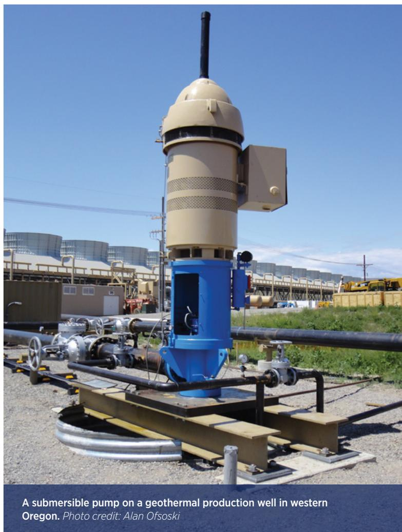
A submersible pump on a geothermal production well in western Oregon. Photo credit: Alan Ofsoski
