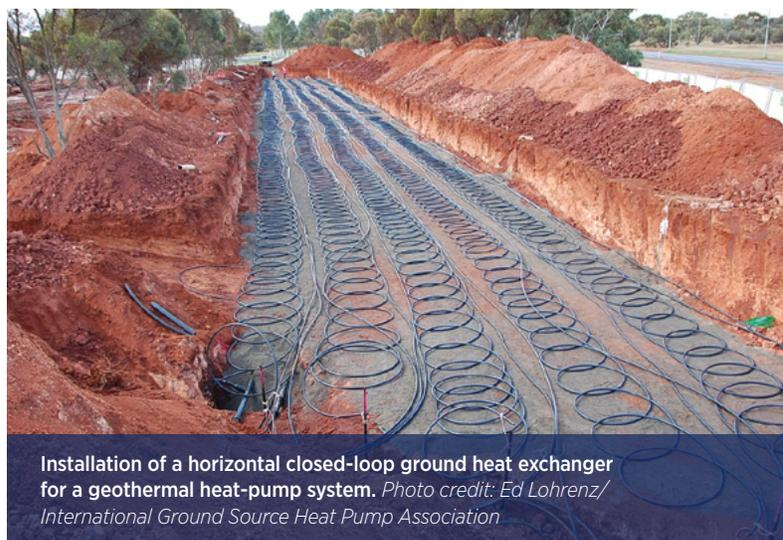
Installation of a horizontal closed-loop ground heat exchanger for a geothermal heat-pump system. Photo credit: Ed Lohrenz/
