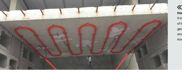
**Keeping Drivers Safe**. Pipe loops spaced 6 inches apart insulate 4,300 square feet of bridge deck. The pipe carries warm, geothermally heated fluid that prevents snow and ice from forming on the bridge. *Photo from University of Texas at Arlington*
