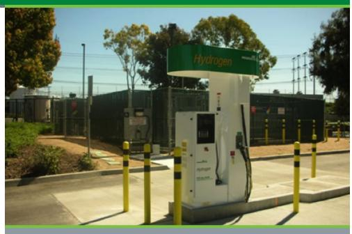
Photograph of the state-of-the-art hydrogen fueling station with fueling at 5,000 and 10,000 psi according to the latest SAE protocols for rapid 3-minute complete tank refueling.
