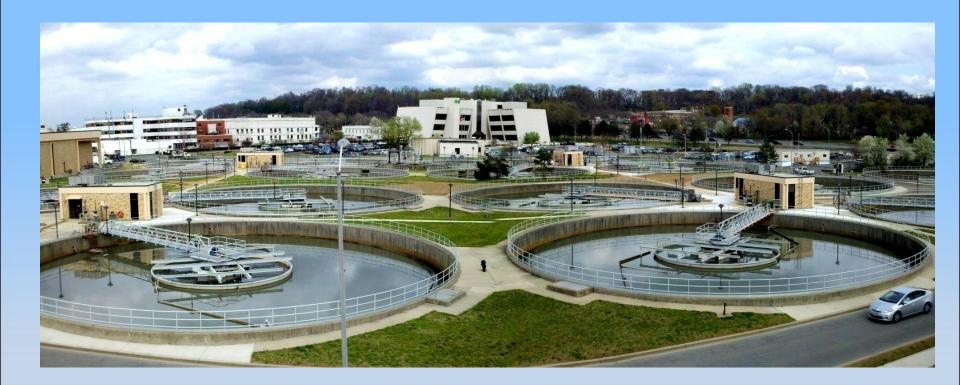
4% ENERGY CONSUMPTION - Removal Of Solids by Settling 35% of CBOD – 50% TSS Ferric Chloride & Anionic Polymer Added
