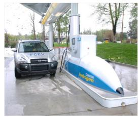
At Chevron's hydrogen station in Chino, California, hydrogen is produced onsite via natural gas reforming.
