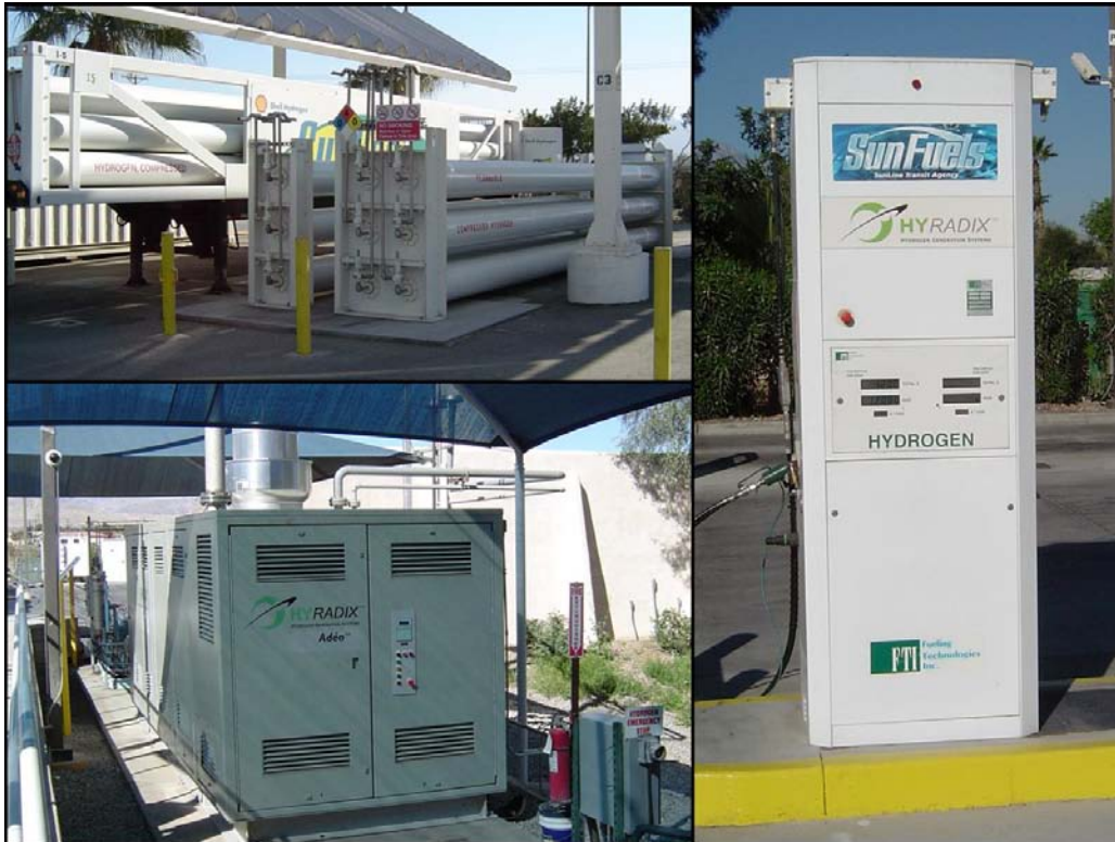
Figure D-6. SunLine's hydrogen storage (top left), HyRadix Adéo commercial reformer (bottom left), and hydrogen dispenser (right)
